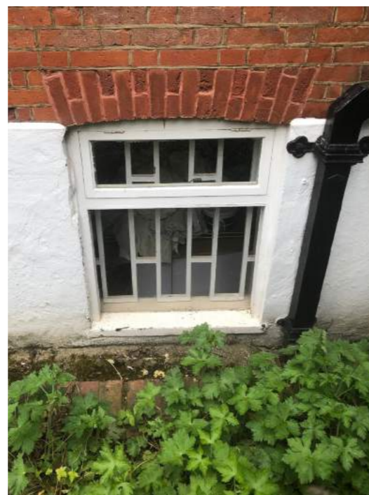
EXISTING WINDOWS IN BASEMENT ROOM
