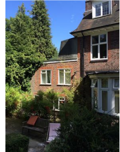
Rear of Side Extension
