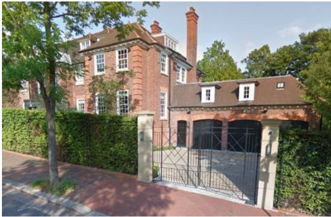
12 Templewood Avenue, NW3 New Front Wing, Side and Basement Pool Extensions
