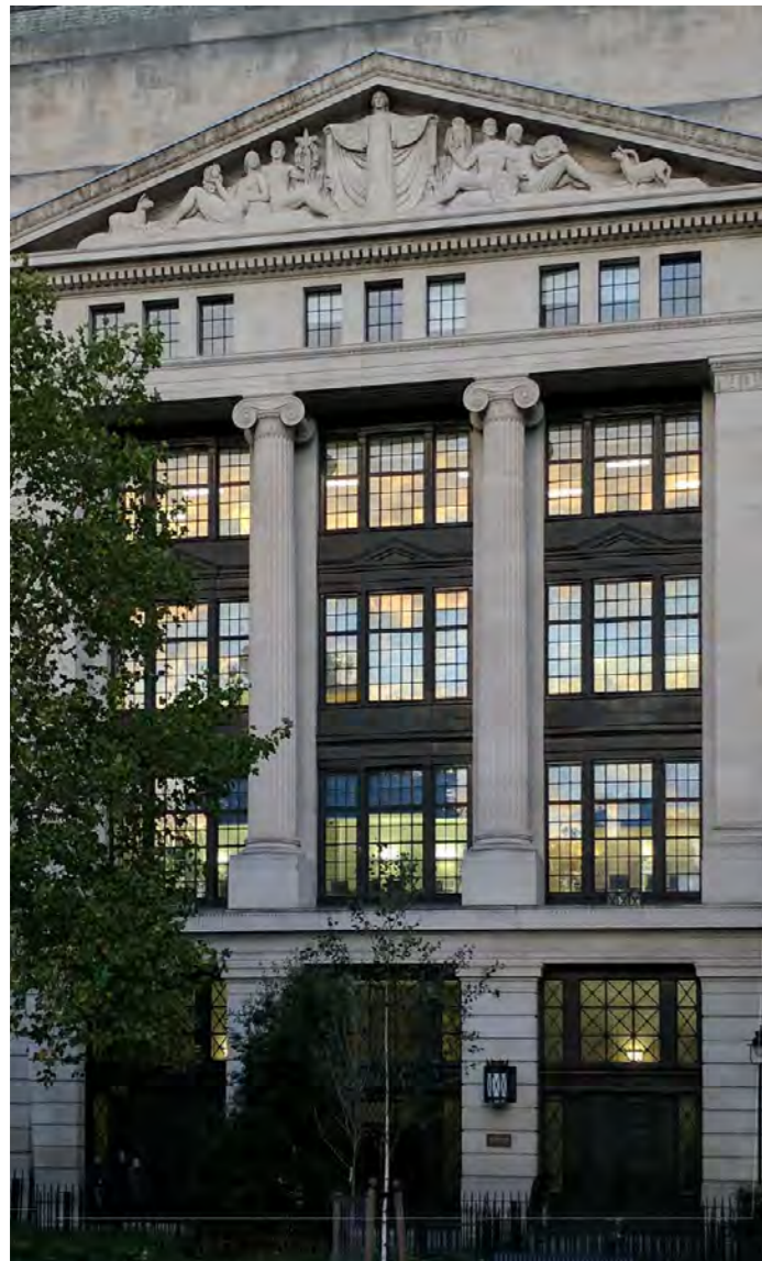
West facade central distyle-in-antis portico
