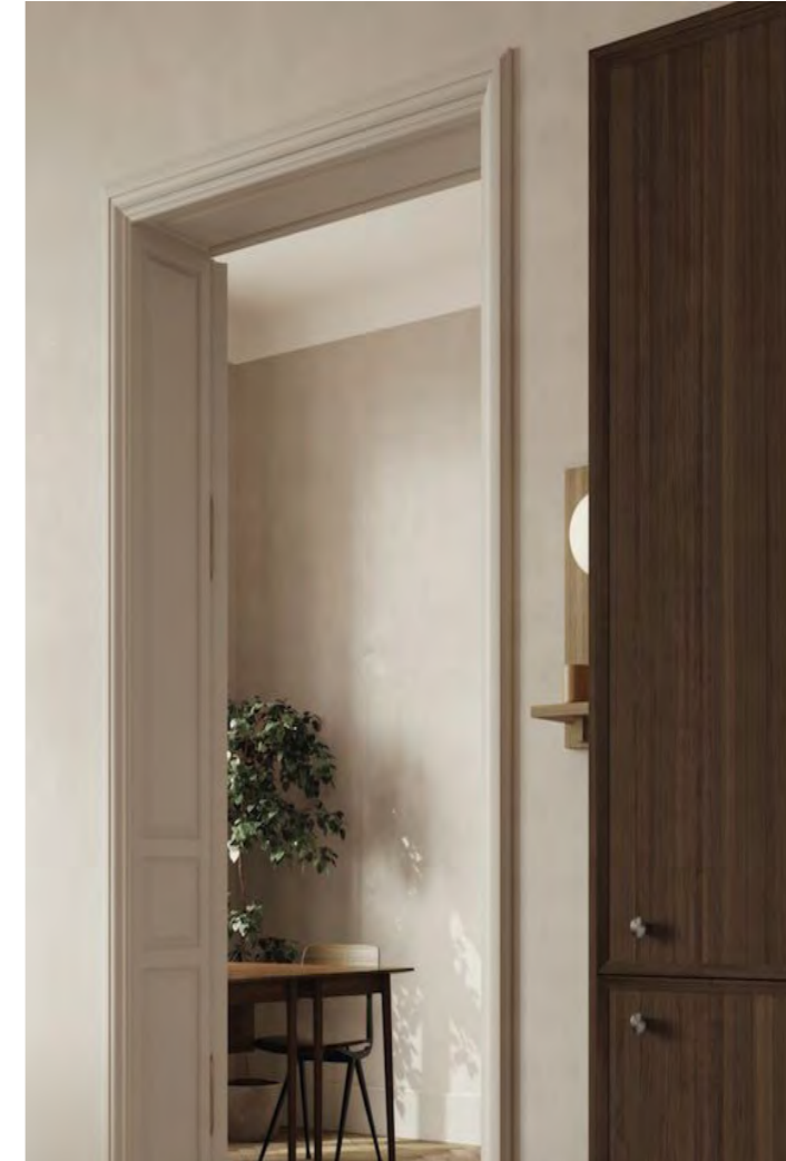
Walls and Ceilings Beams painted RAL 9010 where exposed Ceilings painted RAL9010 (bright white) Walls: warm white, colour RAL 9001
