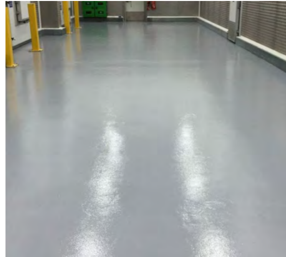
Expoxy Floor Manufacture: Flowcrete Product: Flowcoat SF41 Finish: Mid Grey 280
