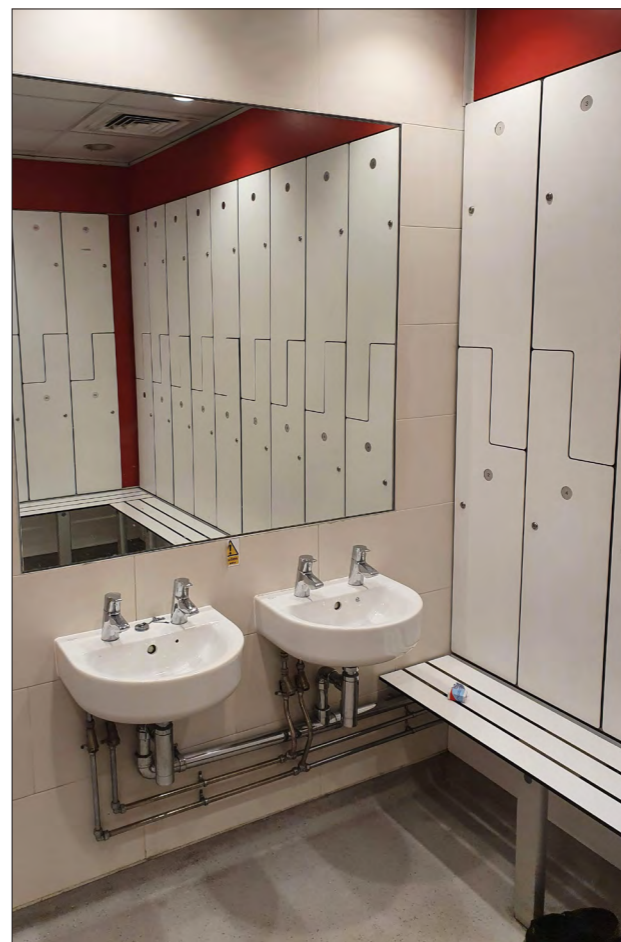
Existing vanity basins to be stripped out
