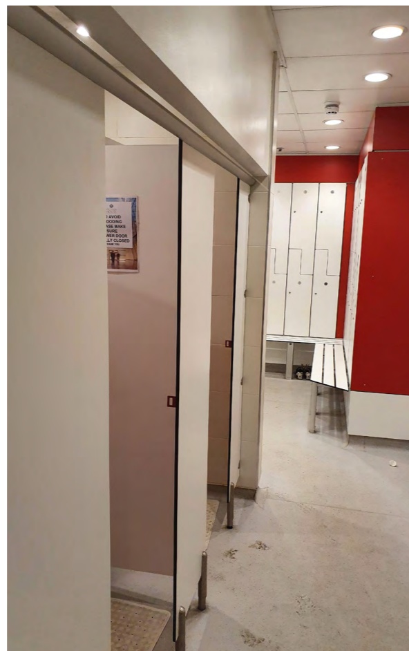
Existing Cubicle System to be stripped out
