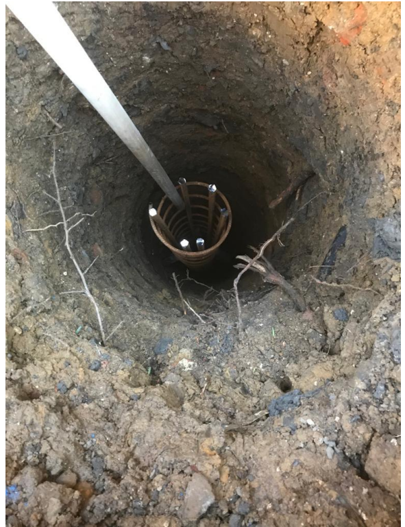
04_Pile + Reinforcement
