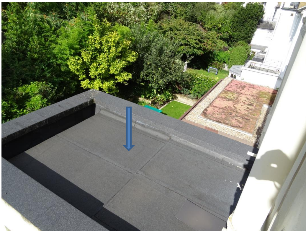
PHOTOGRAPH 4 THE REAR ADDITION ROOF HAS BEEN COVERED WITH ROOFING FELT
