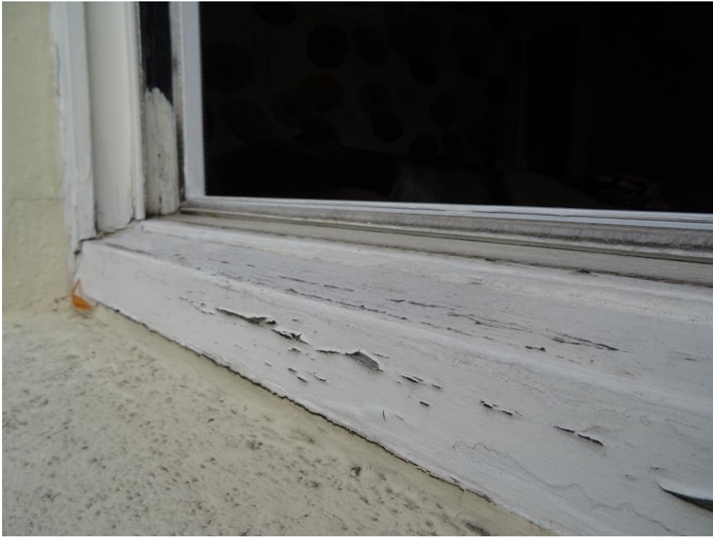
PHOTOGRAPH 27 PEELING PAINT TO THIS WINDOW CILL
