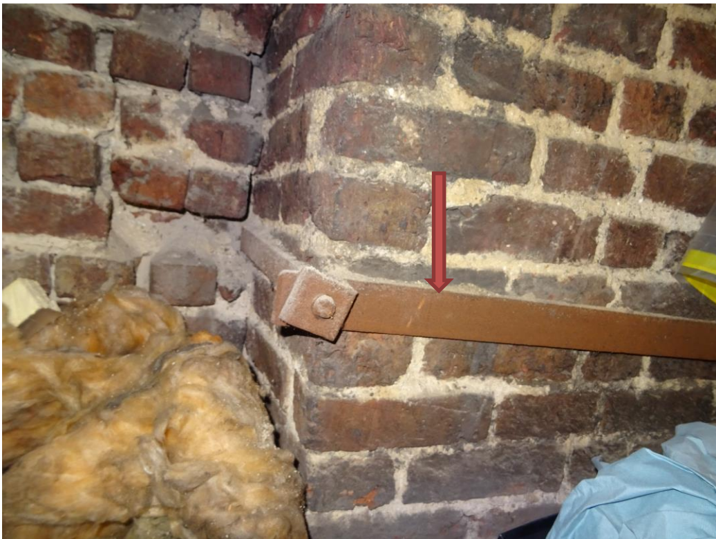
PHOTOGRAPH 16 A METAL TIE TO THE CHIMNEY STACK
