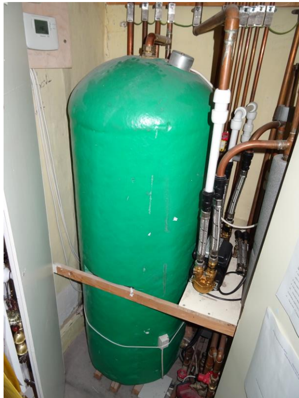
PHOTOGRAPH 28 THE HOT WATER CYLINDER
