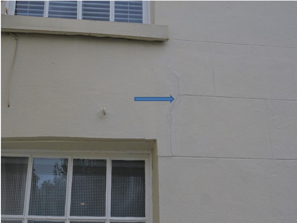
PHOTOGRAPH 21 MINOR CRACKS TO THE REAR WALL
