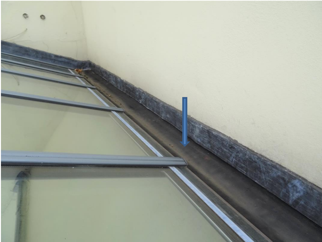
PHOTOGRAPH 7 THERE ARE BOX GUTTERS TO EACH SIDE OF THE CONSERVATORY ROOF
