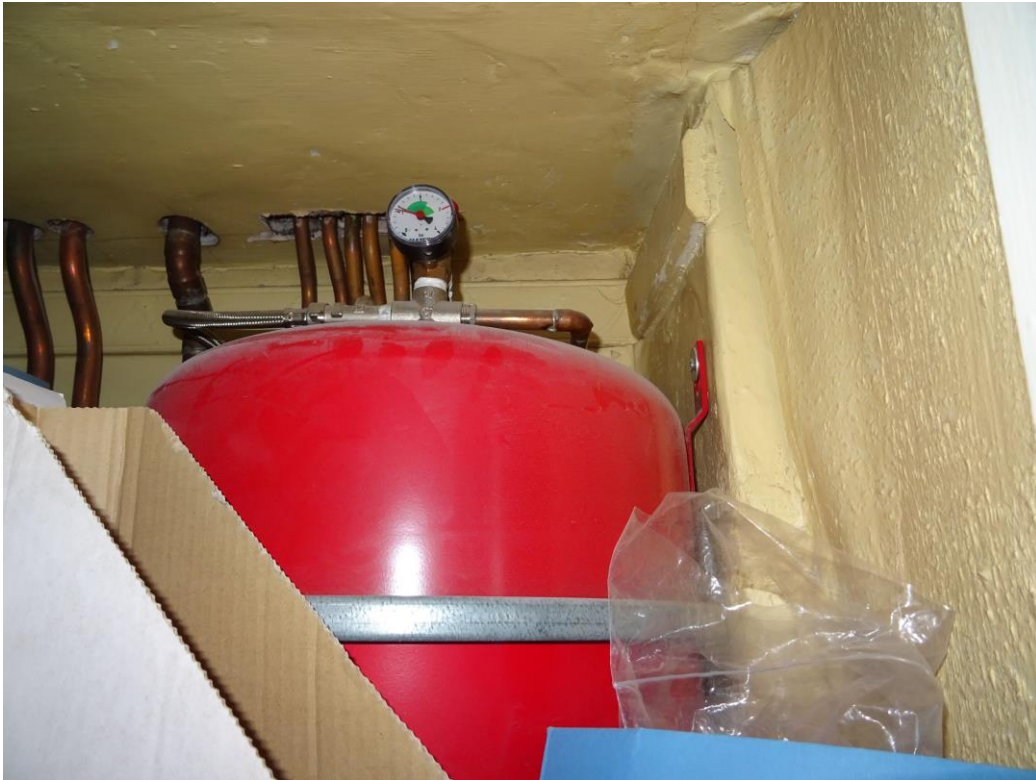
PHOTOGRAPH 29 THE FEED/EXPANSION VESSEL
