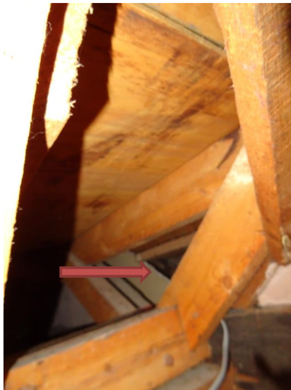
PHOTOGRAPH 14 THERE IS A GAP IN THE RIGHT PARTY WALL BELOW THE VALLEY GUTTER
