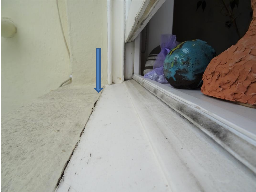
PHOTOGRAPH 31 THE RECEPTION ROOM TIMBER WINDOW SUB-CILL IS FLUSH WITH THE STONE CILL
