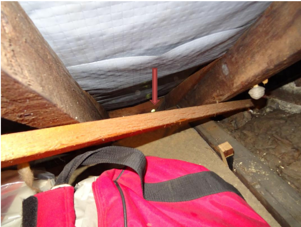
PHOTOGRAPH 17 SMALL HOLES HAVE BEEN PROVIDED TO ALLOW FOR SOME VENTILATION
