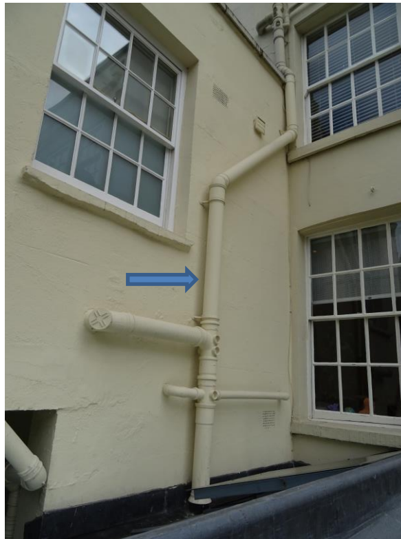
PHOTOGRAPH 3 A PVC SOIL VENT PIPE
