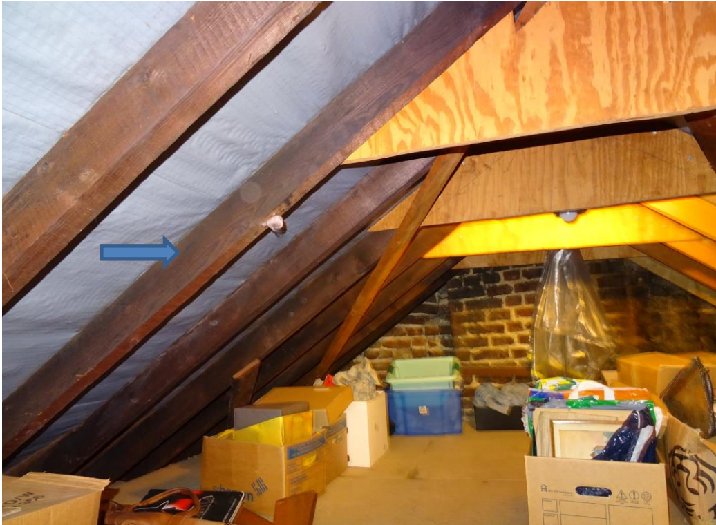
PHOTOGRAPH 13 THE FRONT SLOPE OF THE FRONT PITCHED ROOF HAS THE ORIGINAL RAFTERS
