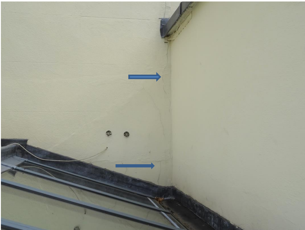
PHOTOGRAPH 20 MINOR CRACKS TO THE REAR WALL
