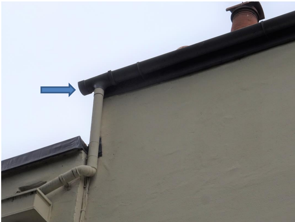
PHOTOGRAPH 2 PVC GUTTER AND RAINWATER PIPE
