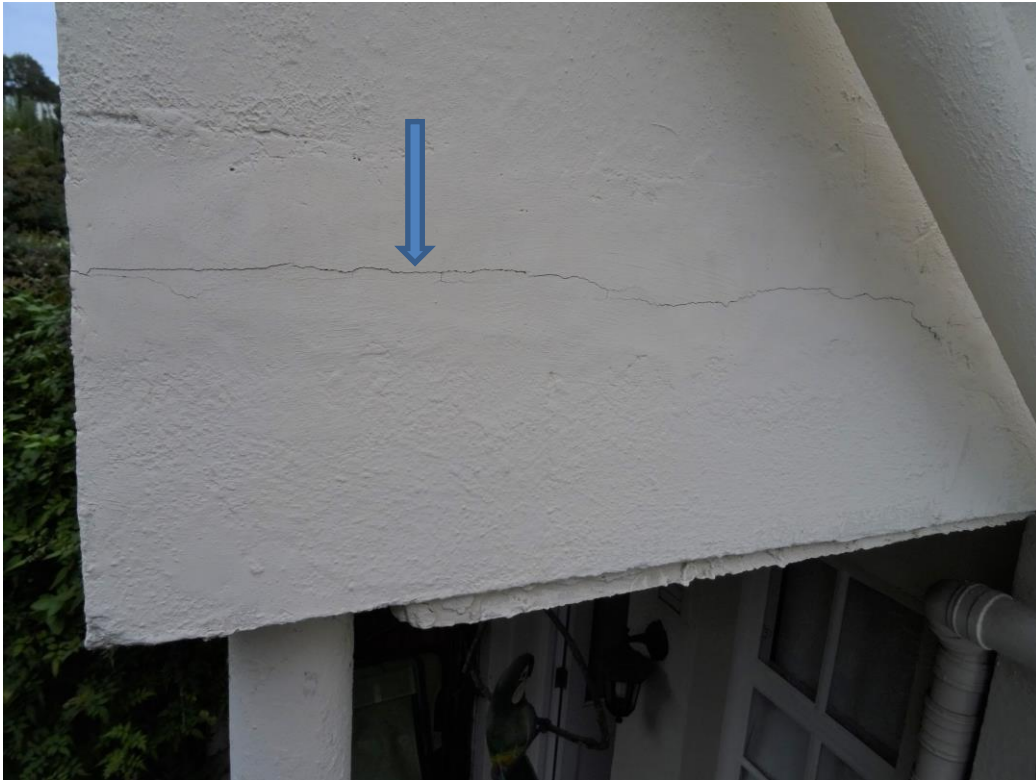
PHOTOGRAPH 25 MINOR CRACKS FOLLOW THE OUTLINE OF THE STEEL FRAME
