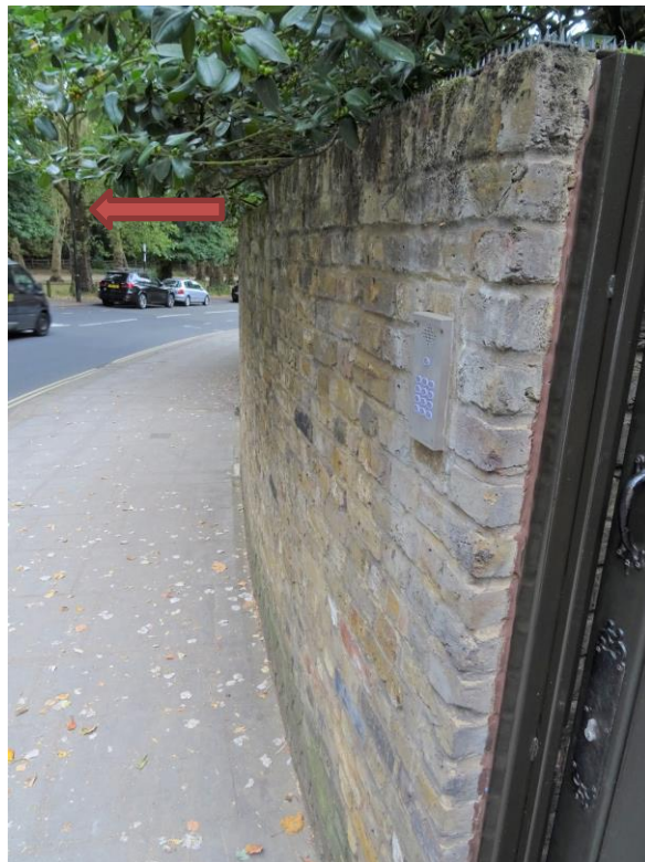
PHOTOGRAPH 30 THE TOP OF THE FRONT BOUNDARY WALL LEANS OUT
