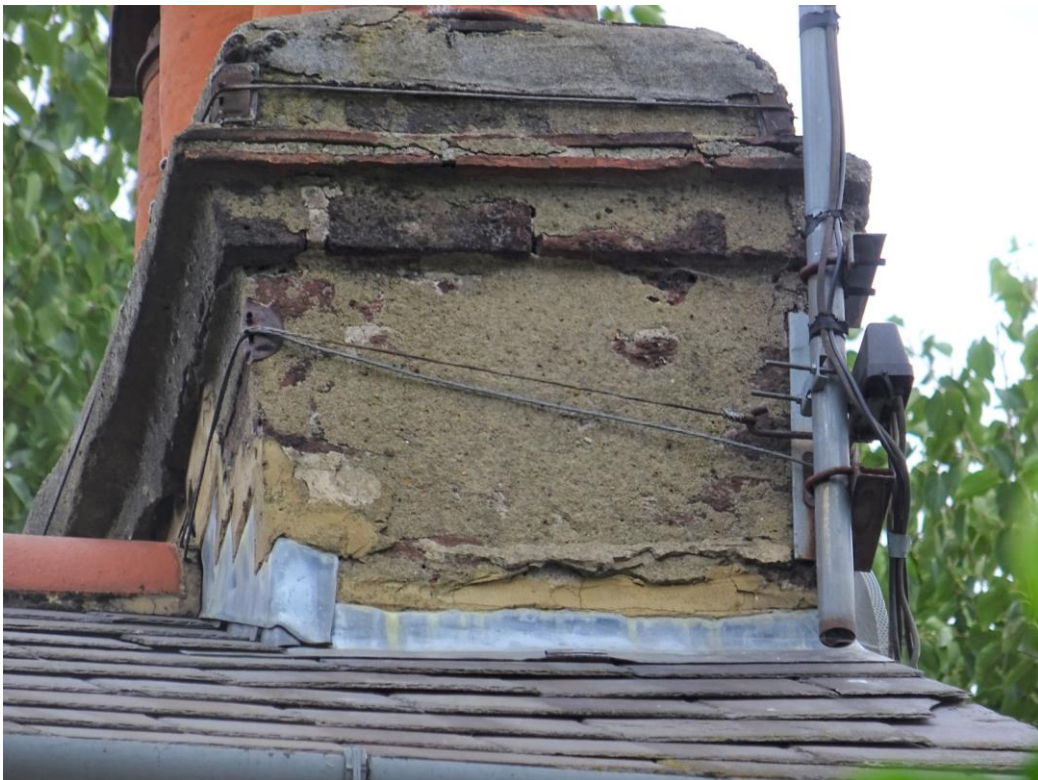
PHOTOGRAPH 10 POOR QUALITY RENDER TO THE CHIMNEY STACK
