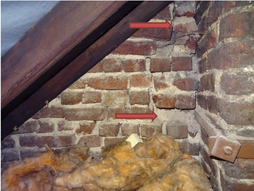
PHOTOGRAPH 15 LOOSE BRICKS TO THE LEFT PARTY WALL
