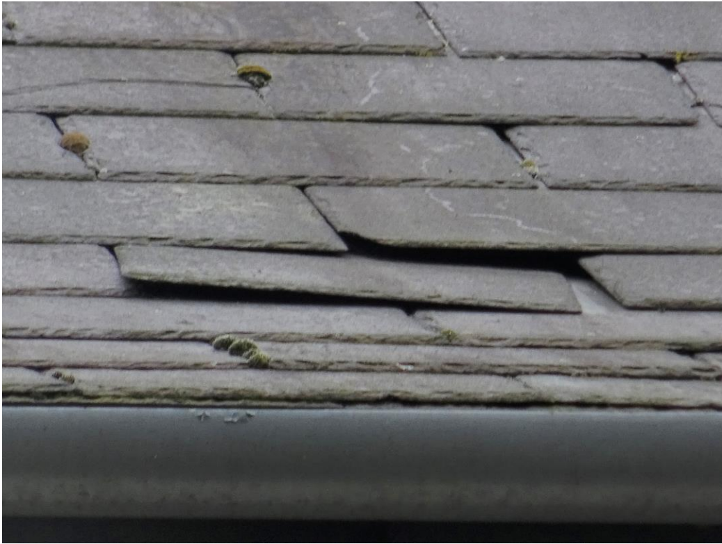
PHOTOGRAPH 5 A LOOSE SLATE TO THE FRONT SLOPE
