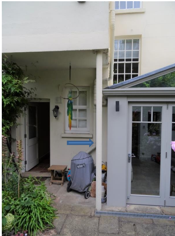
PHOTOGRAPH 23 THE REAR ADDITION IS PARTLY SUPPORTED BY METAL COLUMNS
