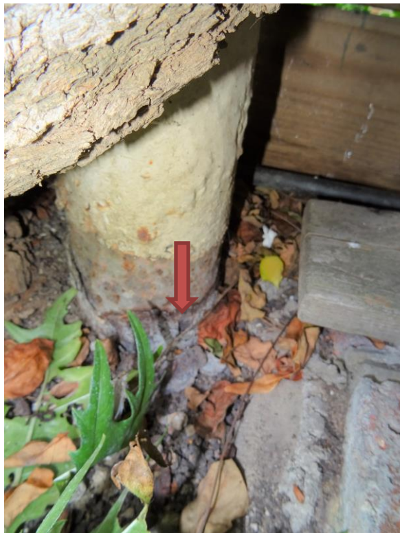
PHOTOGRAPH 24 THE BOTTOM OF THE COLUMNS ARE CORRODING
