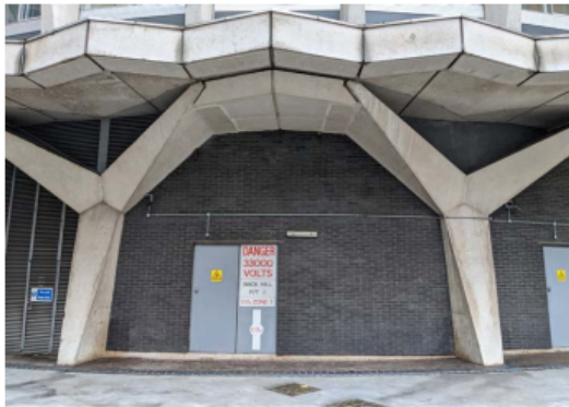
Site photo - existing 33kV UKPN substation transformer bay
