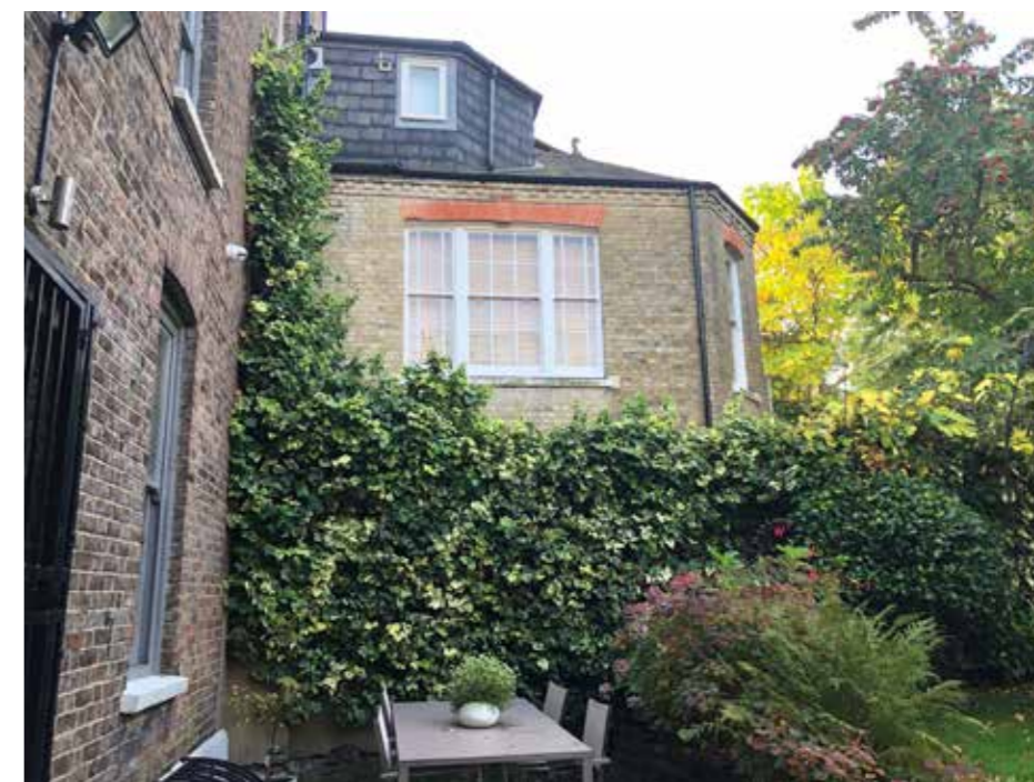
Figure 4.7 The back of No. 7 Pilgrim’s Lane has been altered dramatically over its lifetime.
