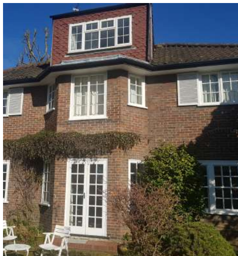
(photo showing rear dormer window)
