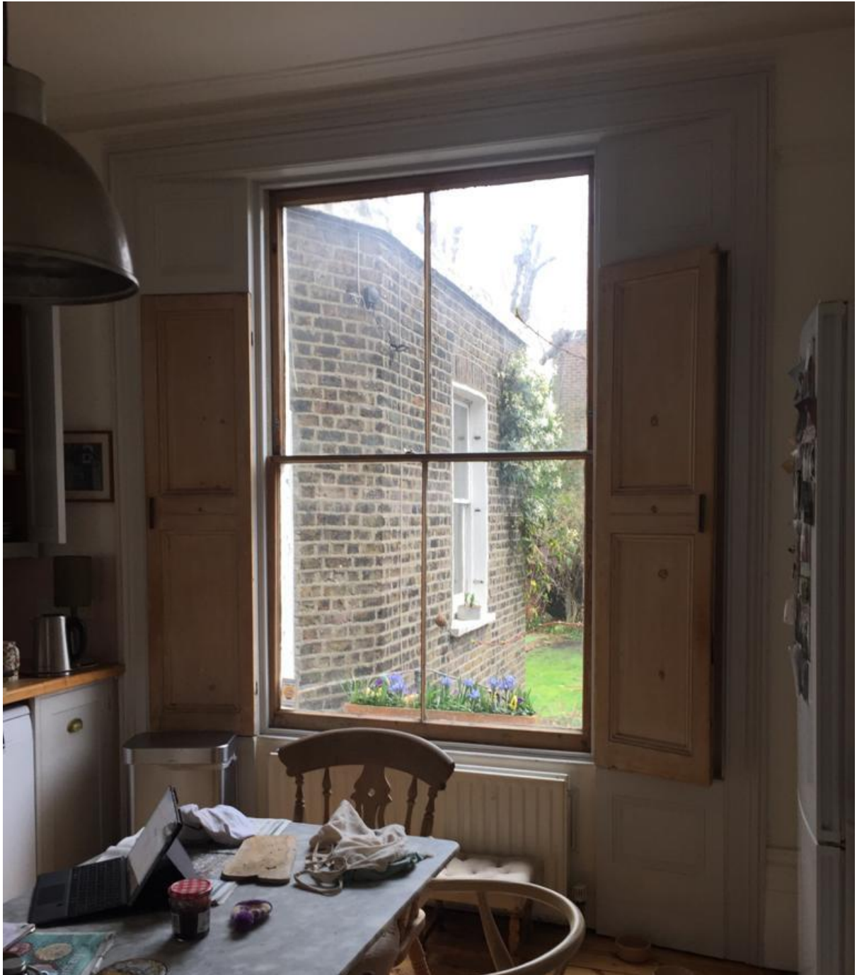
Internal view of existing double hung timber sash unit
