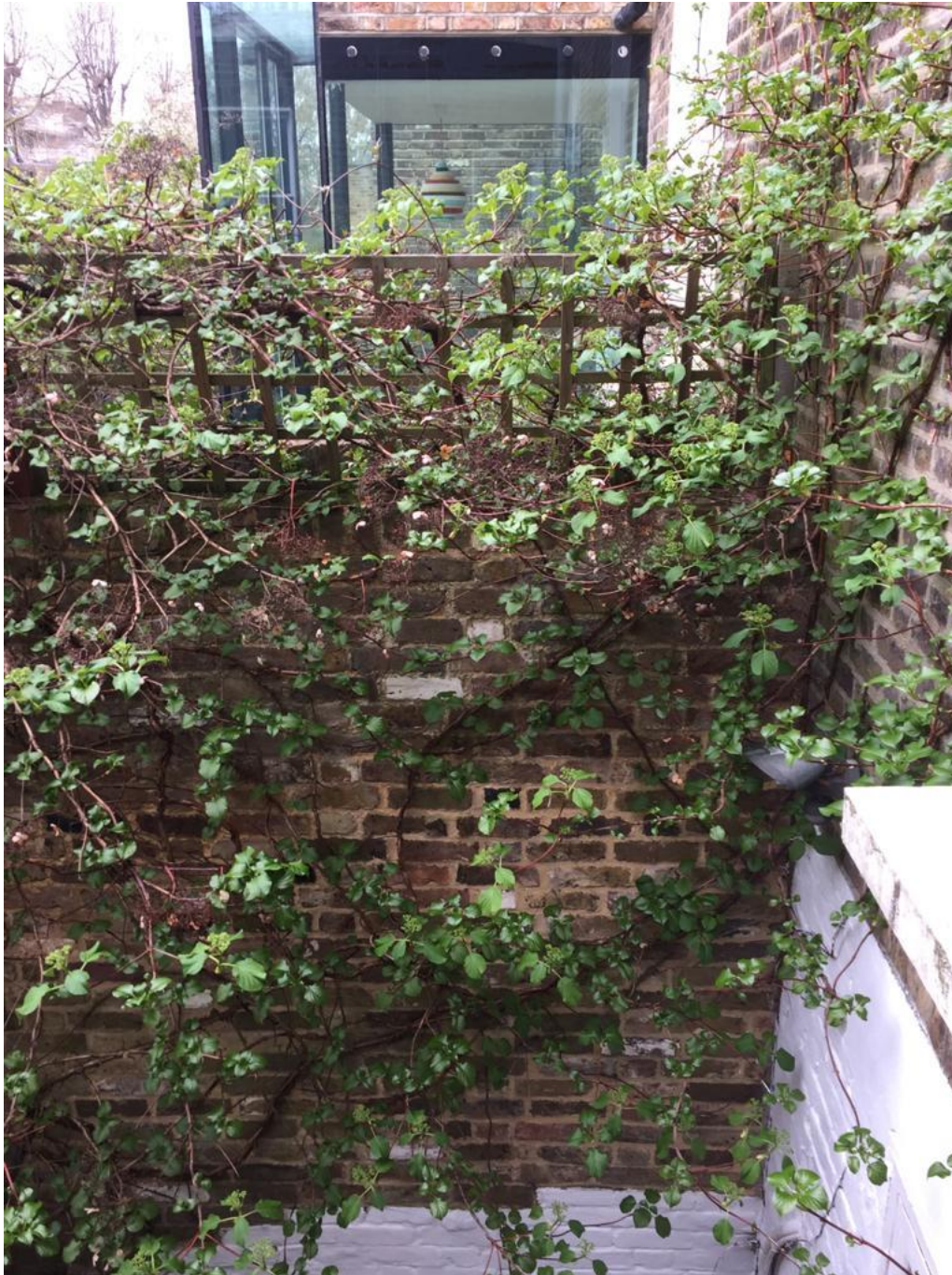
View of party wall from existing external stair access
