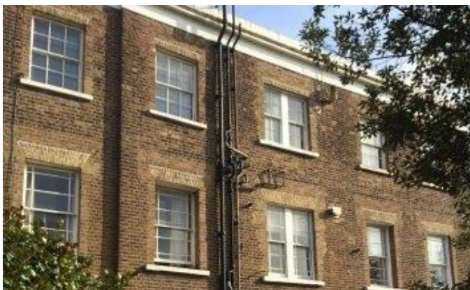
Fig 8: Contrast between window style and lintels
