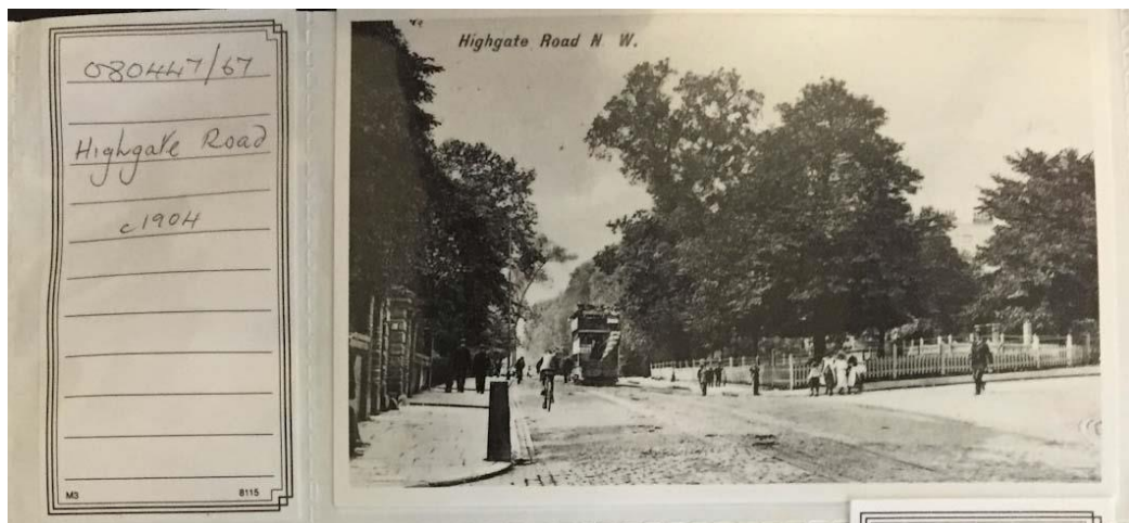
Fig 6: Photograph of Highgate Road showing Grove End House between the trees on right
