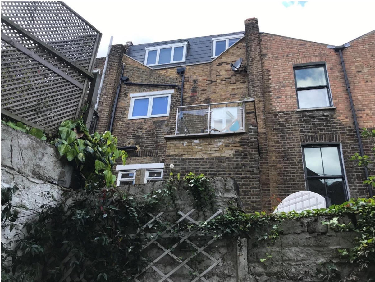
13 Healey Street with second floor terrace and third floor mansard roof extension, as seen overlooking the garden of 13 Grafton Crescent. The first-floor terrace at 14 Grafton Crescent, one of three roof terraces to that property, is also visible at left.
