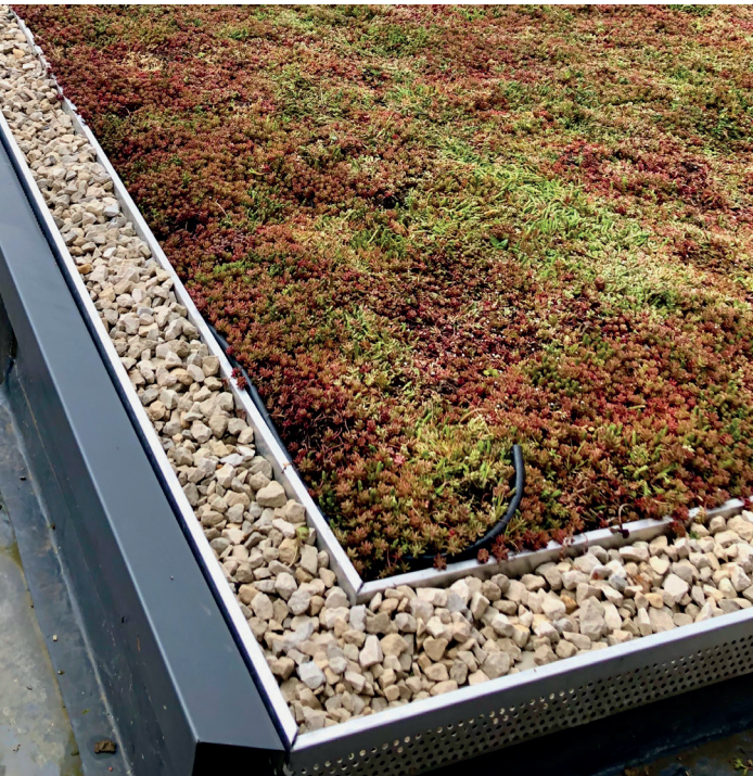
Aluminium angle profiles for retaining material in the absence of parapet, and for separating vegetation from pebbles
