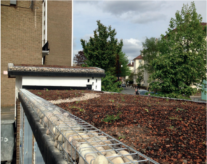
Galvanised gabion with pebble infill provides a beautiful counterpoint to the planting and habitat features
