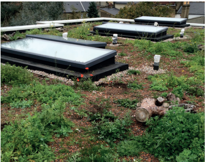
Arrangements of natural materials to add visual interest and ecological function to the green roof vegetation
