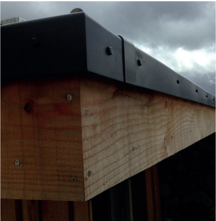
Where necessary your waterproofing can be finished with a graphite plastic trim to provide a drip edge or simple finish
