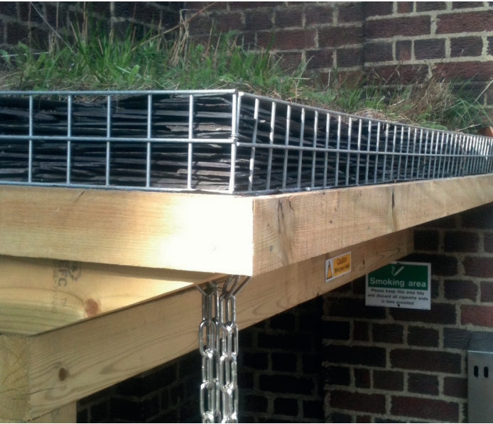
Gabion can also be installed with reclaimed slate. This smoking shelter also features a rainchain to carry water to the ground
