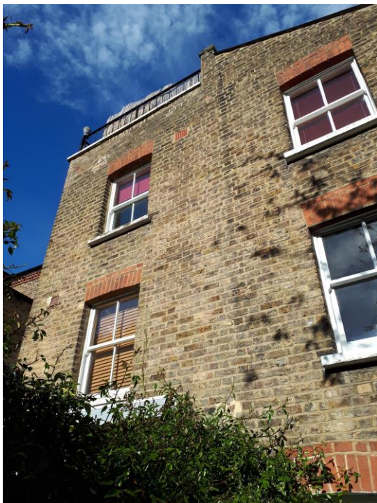
Existing view towards no 45 rear
