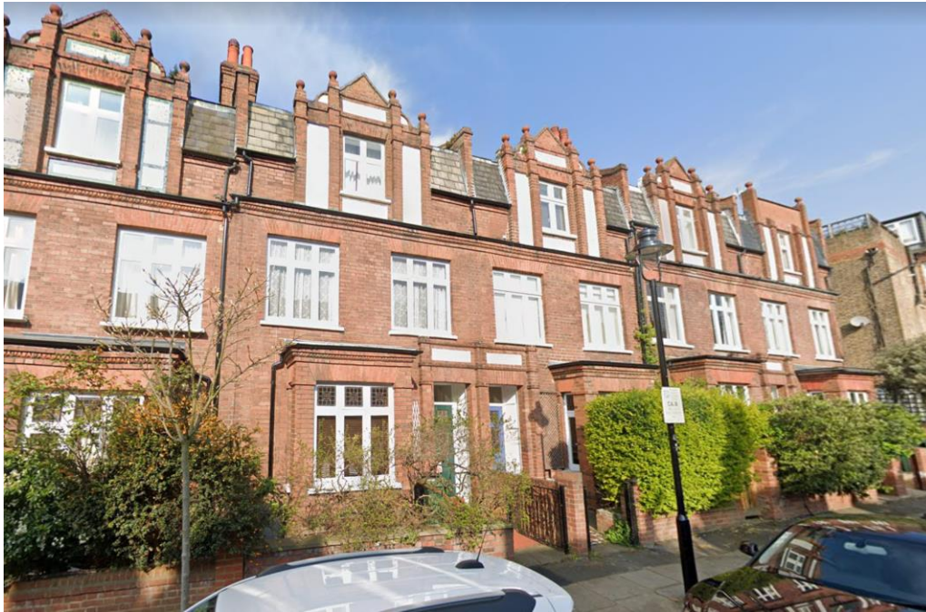
View from Lisburne Road
