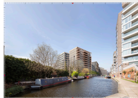
5 | Regent's Canal Towpath, looking north
