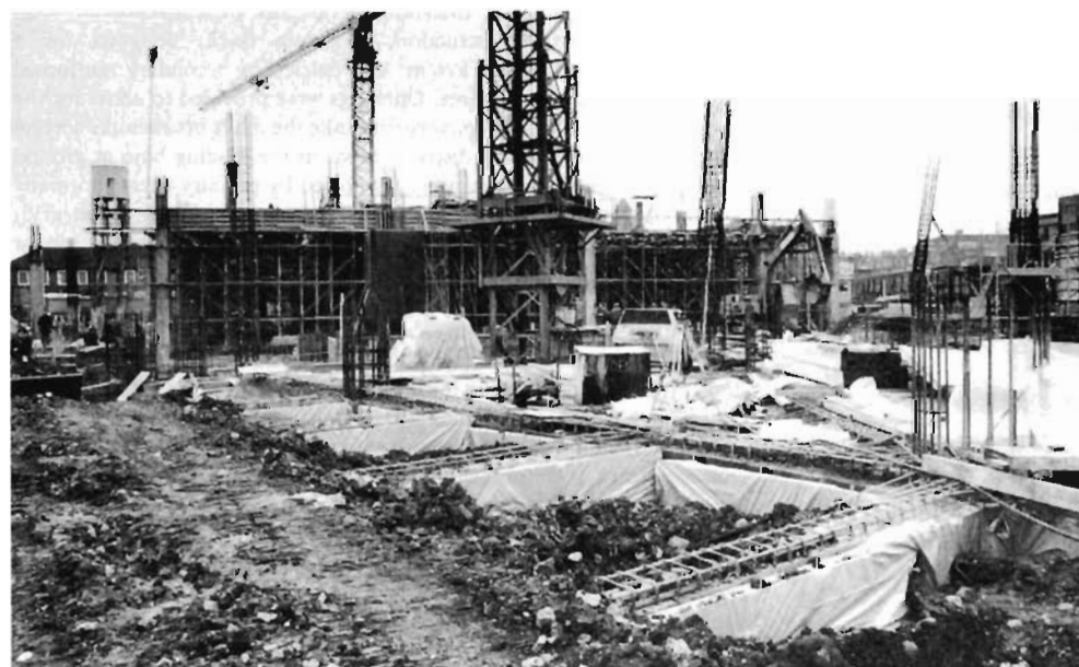
Fig 9. Clayboard protection to ground beams
