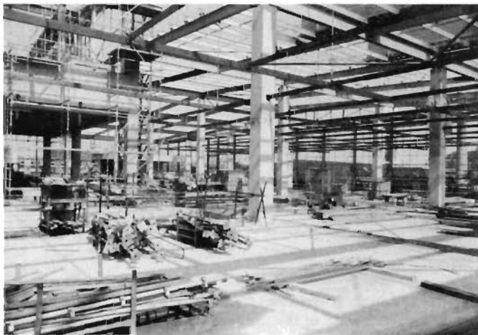
Fig 12. Services subframe in the sorting office
