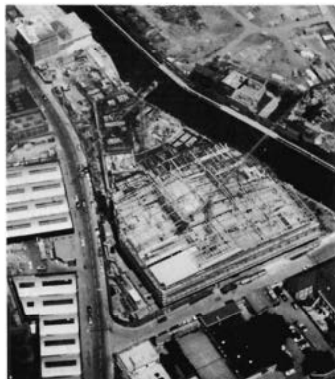
Fig 14. Aerial view—superstructure in progress
