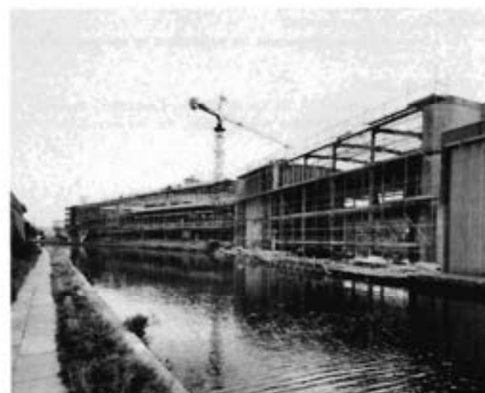
Fig 13. Canal elevation structural frame nearing completion
