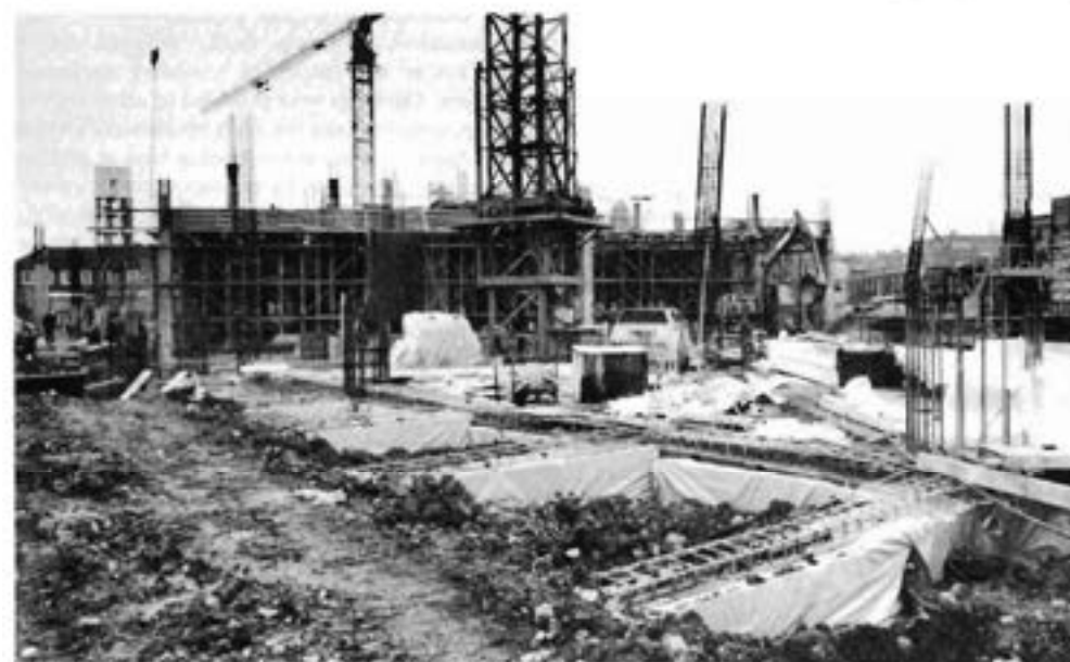
Fig 9. Clayboard protection to ground beams
