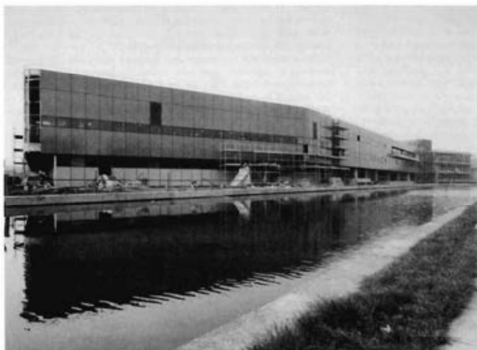
Fig 11. Canal elevation cladding nearing completion
