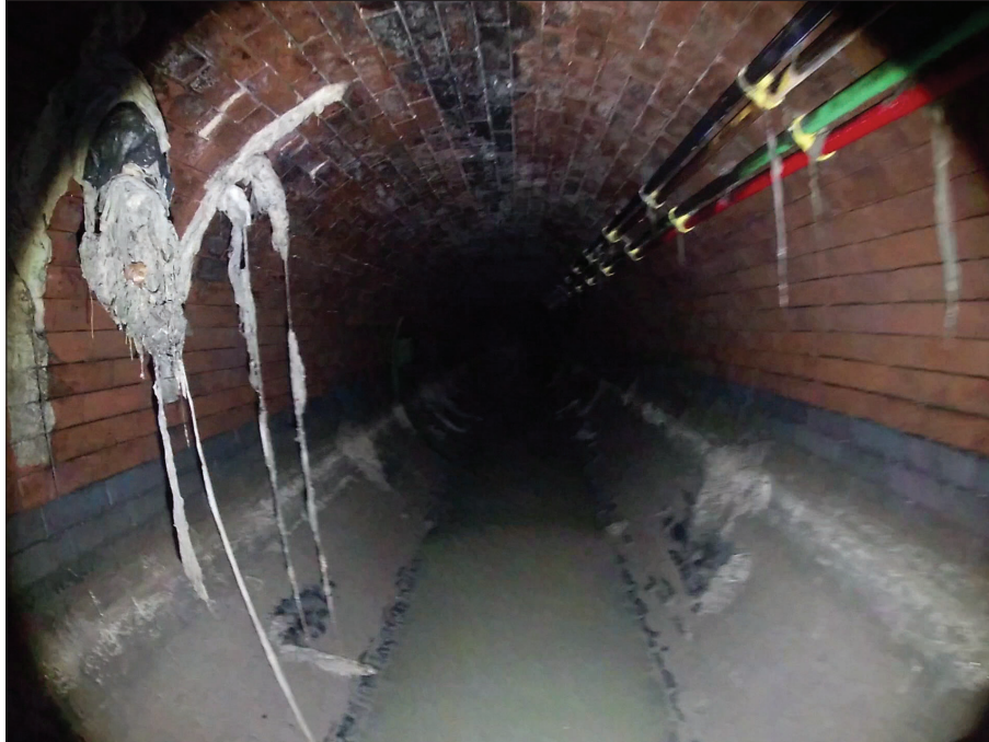
Photo: TQ29835701_D_150619_233500_-_7.jpg, Media No.: 42774, 00:04:01 93m, Attached deposits, encrustation, from 9 to 11 o'clock, 10% cross-sectional area loss
