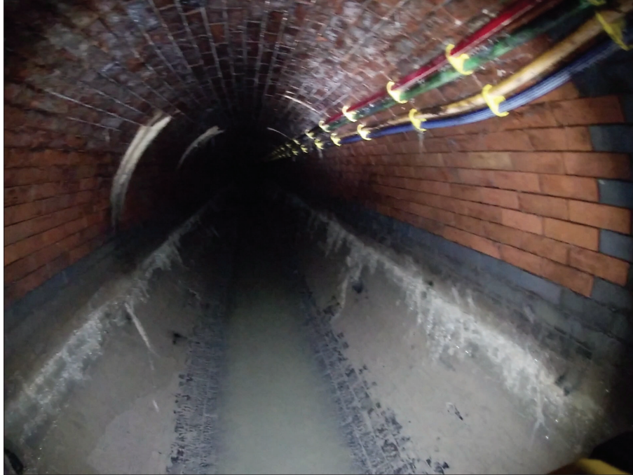
Photo: 1_1_5_A.jpg, Media No:: 42774, 00:00:02 0.9m, Attached deposits, grease, from 4 to 8 o'clock, 5% cross-sectional area loss, Start Remarks: PATCHY
