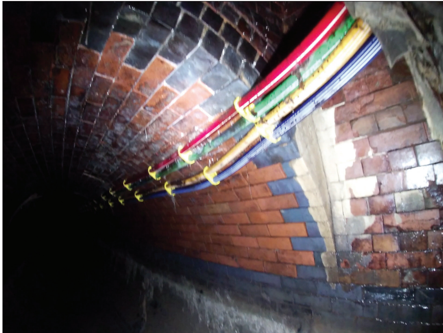
Photo: 1_1_6_A.jpg, Media No:: 42774, 00:00:02 0.9m, Other obstacles, external pipe or cable, from 2 to 3 o'clock, 5% cross-sectional area loss, Start Remarks: CABLES
