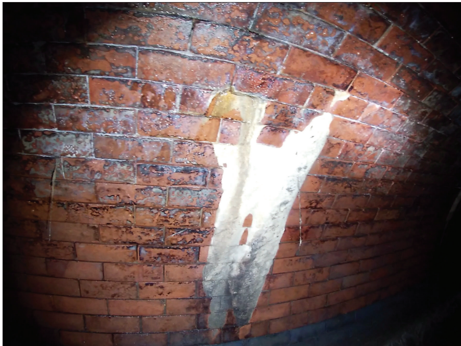
Photo: 1_1_23_A.jpg, Media No.: 42774, 00:00:19 2m, Attached deposits, encrustation, from 8 to 11 o'clock, 5% cross-sectional area loss
