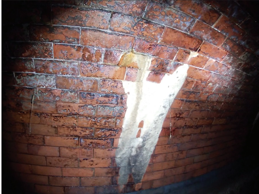
Photo: TQ29835701_U_210619_075829_-_1.jpg, Media No.: 42774, 00:00:19 2m, Infiltration, seeping, from 10 to 11 o'clock
