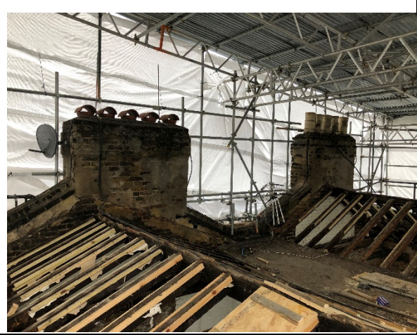
View across roof. Note condition of ridge beam and evidence of previous unsuccessful strengthening measures.
