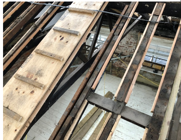
Example of timbers that have been cut into shorter lengths and then fixed back together.
