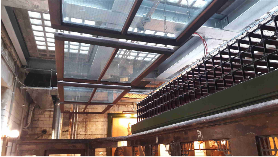
Internal views of the refurbished interior.
