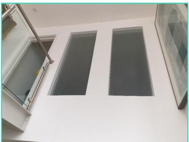
The main window serving the LKD spans the full width of the property and is full height from the ground floor level. It measures 3.9m x3.6m and serves the LKD which is predominately 3.5m deep although a small area increases to 4.5m. The window is therefore almost as tall/wide as the room is deep/wide and in that regard, is a particularly generous window size for this room dimension.
