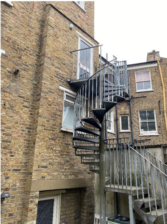
View of existing walkway and stair
