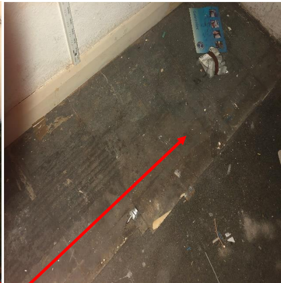
Asbestos Thermoplastic Floor Tiles with Asbestos Adhesive Backing(s) – See Recommendations
