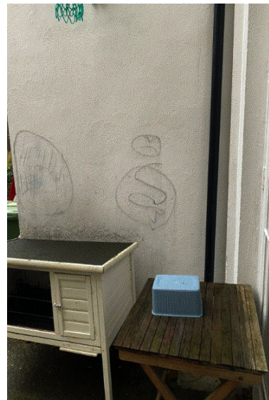
Image 11: Existing wall where proposed WC window to be reintroduced.
