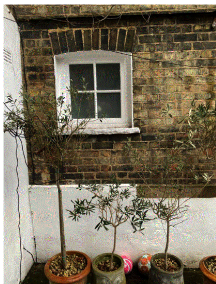
Image 12: Existing window at no.11
