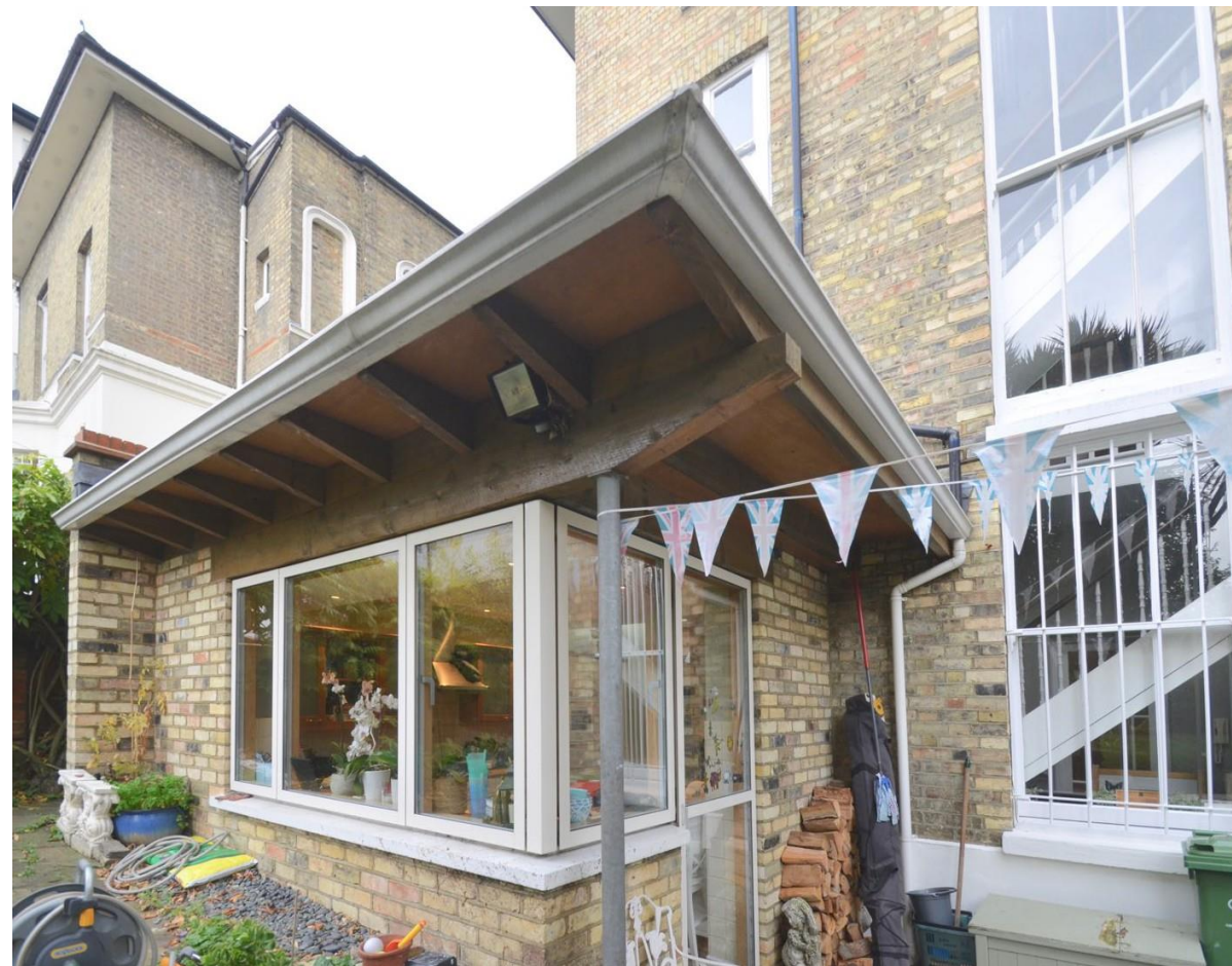
Image 7: Existing non-historic single storey extension
