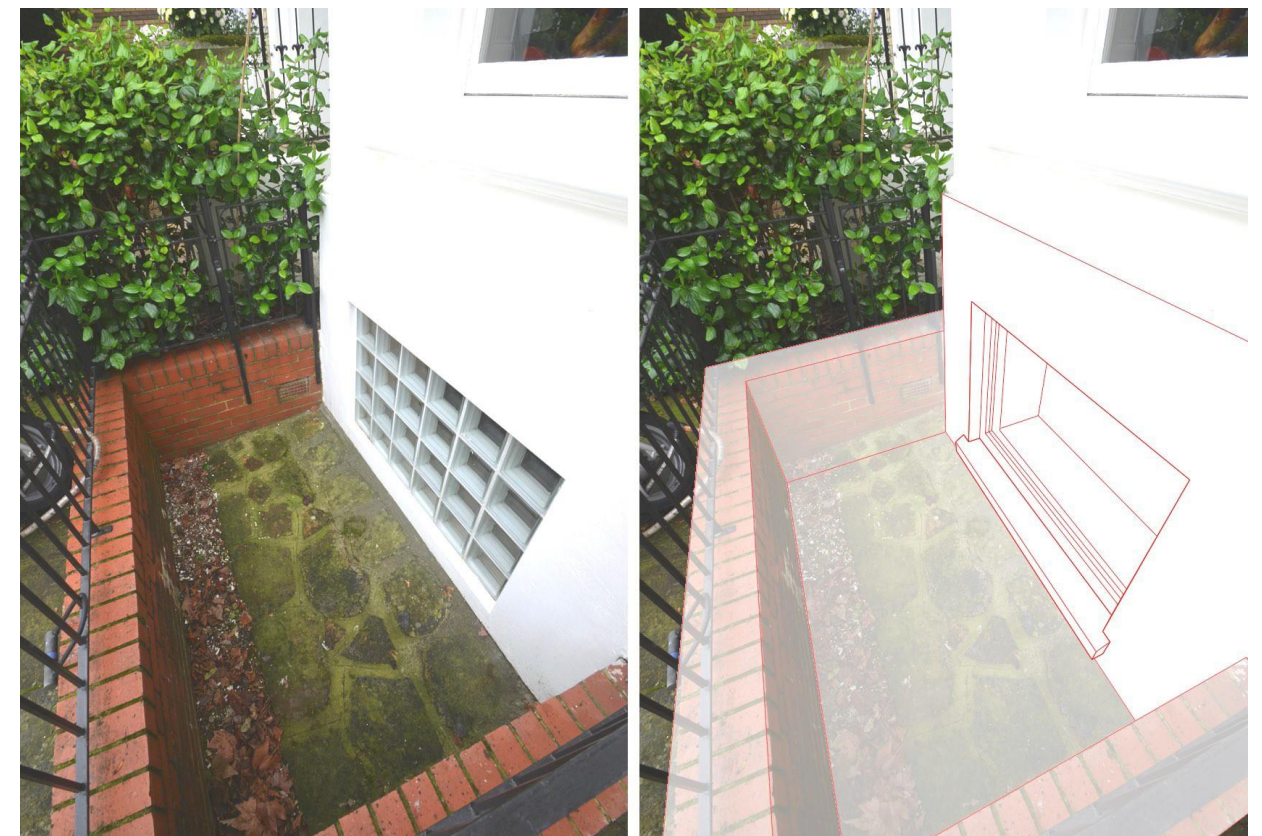
Image 3: Proposed lightwell base & window sill lowered. Walls rendered to match house. New painted timber window with stone cill.
