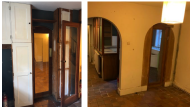
kitchen infill photographed prior to unauthorized removals 2019
