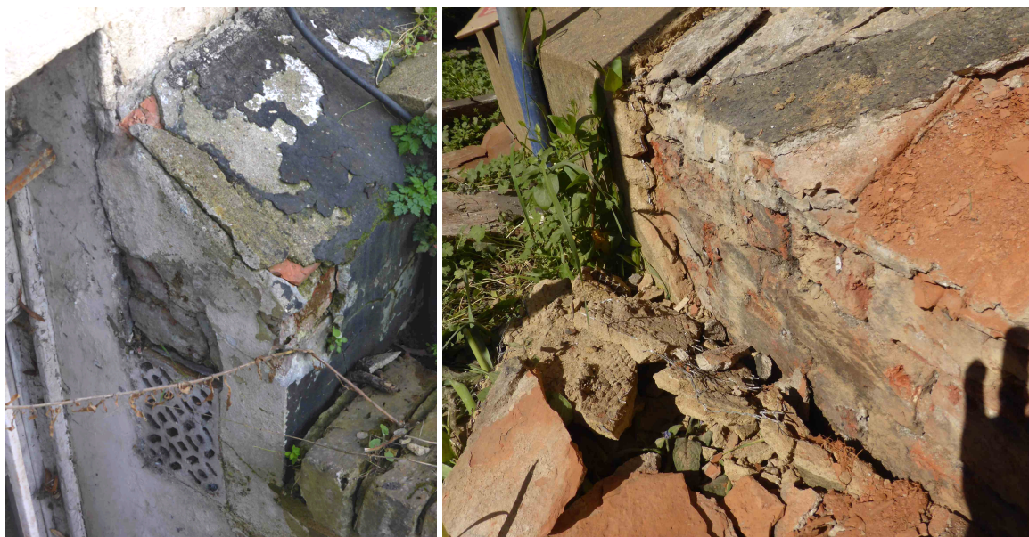
Fig. 1 West wall lightwell showing vented plinth detail
