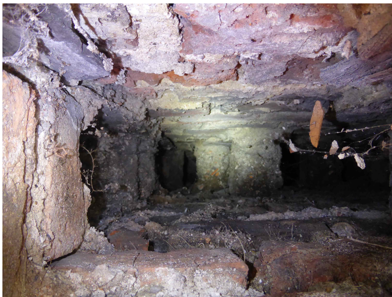
Fig. 3 View down into the vented cavity showing staggered brick stretcher ties
