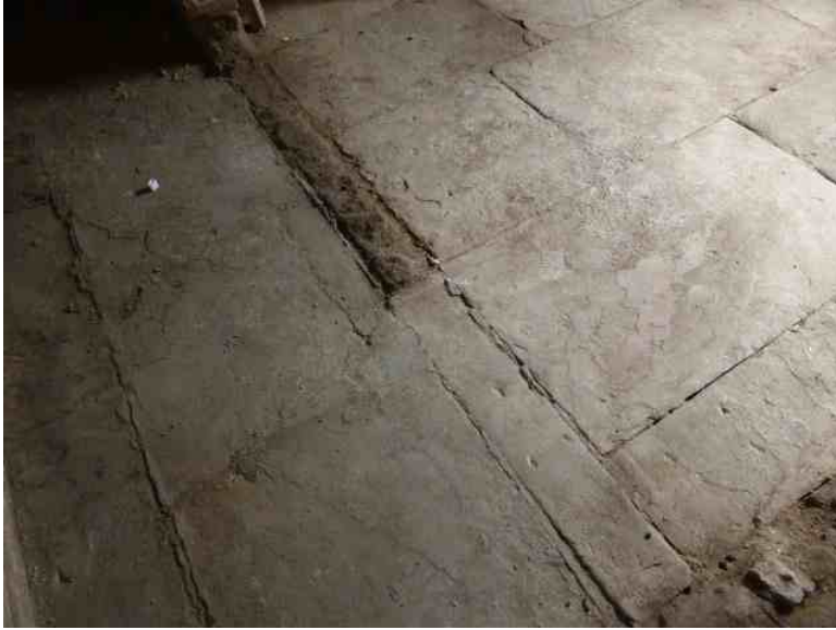
Fig. 4 Uncovered flagstone floor showing original threshold between hallway and scullery
