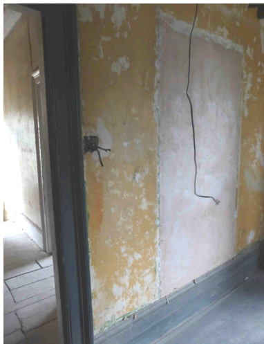
Fig. 8 Gypsum plaster door infill to be retained as found
