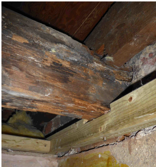
Fig. 9 Underside of the valley beam at bearing point on masonry wall
