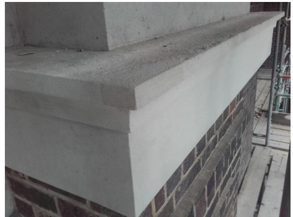
Repair and repointing to corner of stone cornice.
