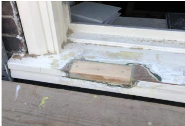
Splice repair to window sill with oak timber to lower ground window.
