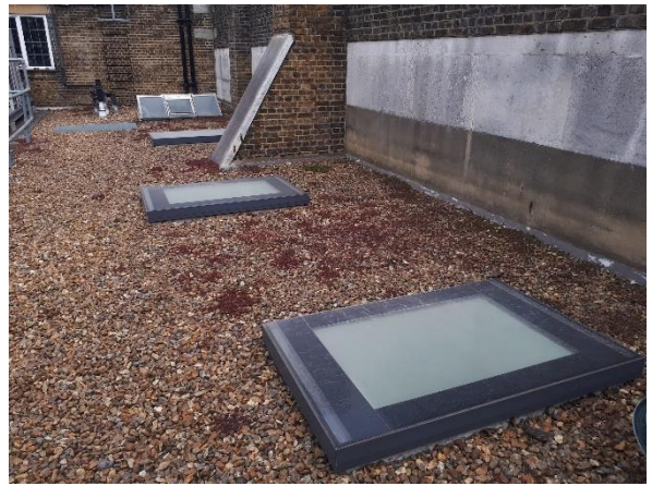
Modern roof lights within Roof 4. We propose to replace the lantern roof light to match.
