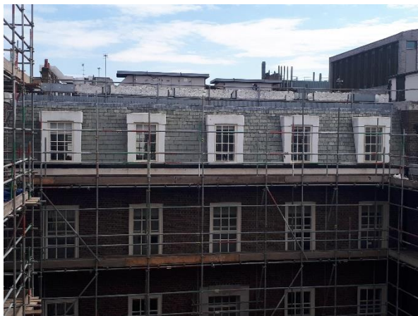
View of window surrounds to mansard roof within internal courtyard.
