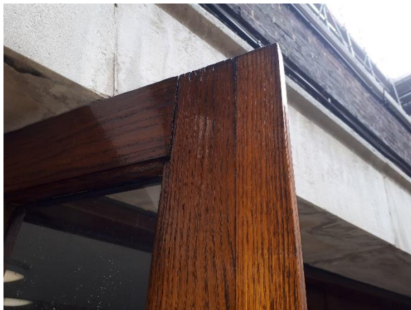
Example of open joint to existing oak door set within the internal courtyard.
