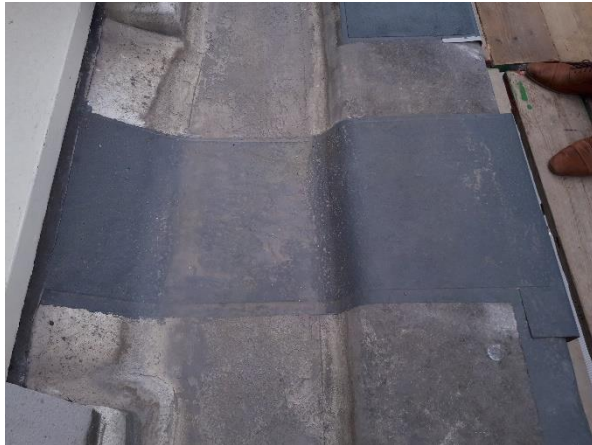
Sample of overlay on existing asphalt cornice with a cold applied liquid system.
