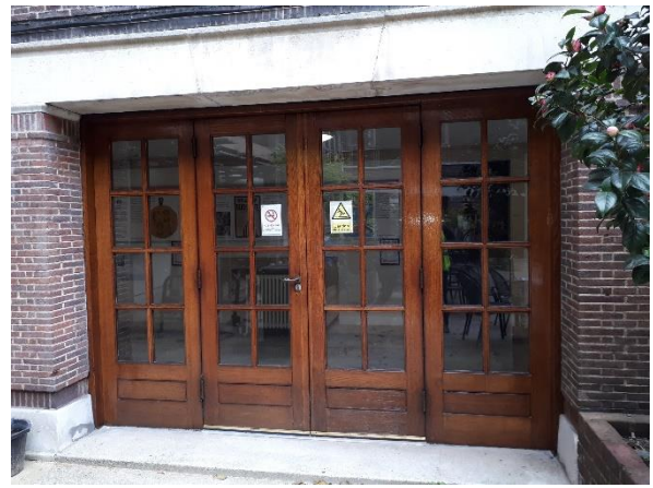
Photograph showing the configuration of door sets within the internal courtyard.
