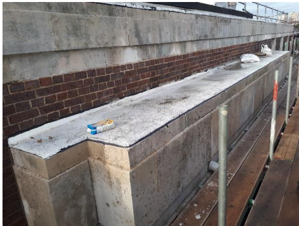
Existing asphalt finish on cornice above portico on garden elevation.
