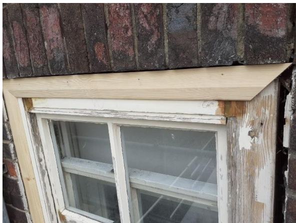
Replacement of softwood architraves to sash window.
