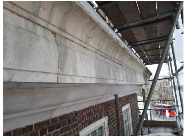
Cleaned stonework to front face of main cornice.
