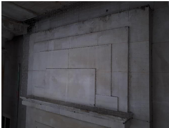
New bird netting installed above main entrance fixed to existing eye hook fixings.
