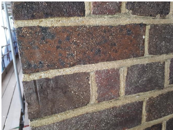
Existing pointing to external elevation.
