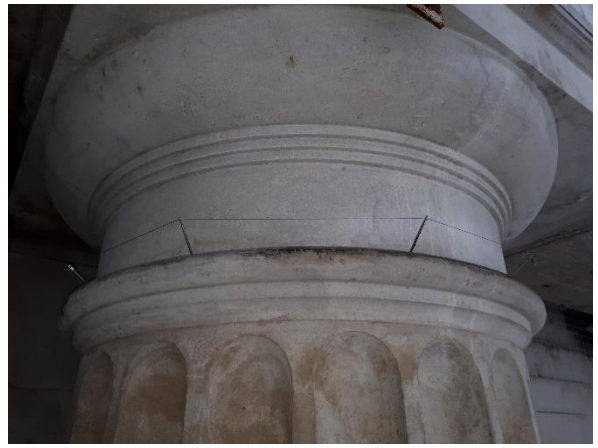
New bird wire to column ledges fixed to existing posts.
