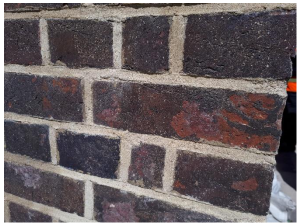
New pointing to external elevation.
