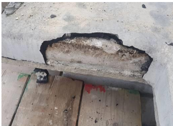
Photo showing thickness of existing asphalt to be removed and stonework under (if the liquid system is not supported).
