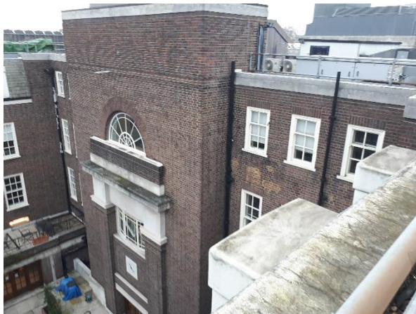
Existing asphalt finish to brick edge detail below semi-circular window within the courtyard.
