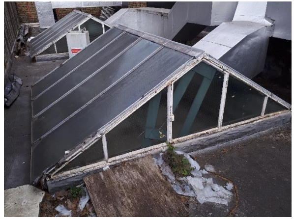
Close up view of roof lights to be removed within Roof 1.
