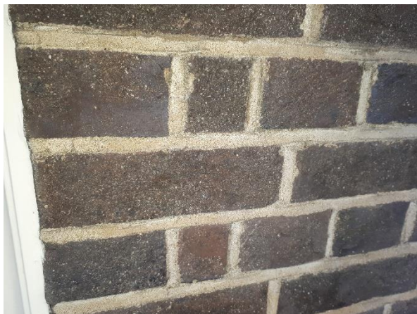
Existing pointing to external elevation.
