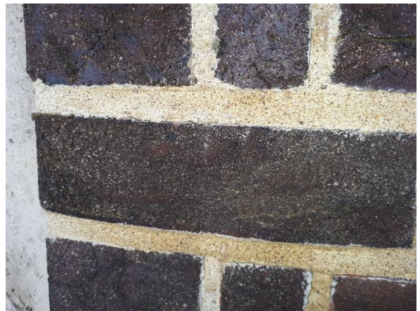
New pointing to external elevation.
