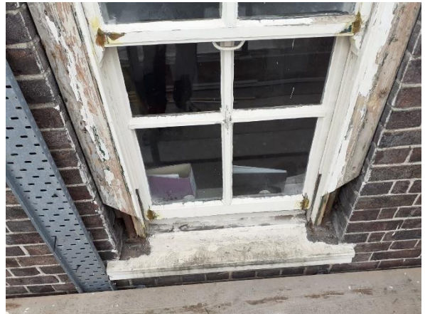
Splice to softwood frame surrounding sash window to remove decayed timber.
