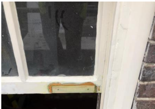
Replacement of decayed bottom rail on sash window with pine timber.
