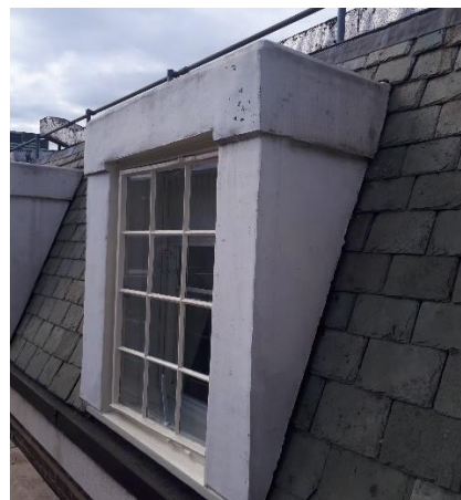
Close up of window surround to mansard roof within internal courtyard.
