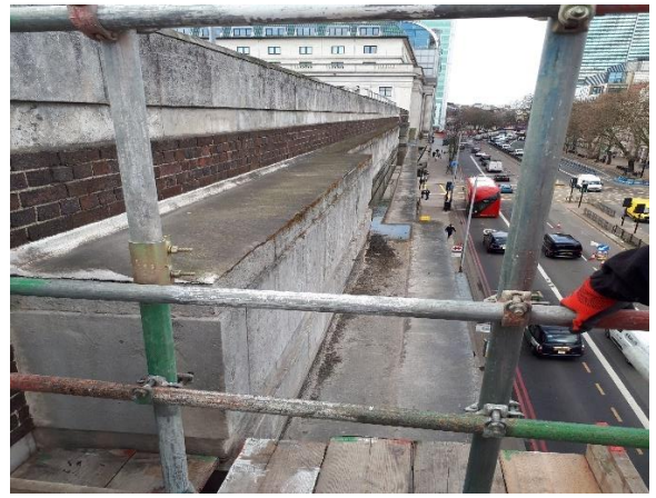
Existing asphalt finish on cornice above portico on Euston road elevation.
