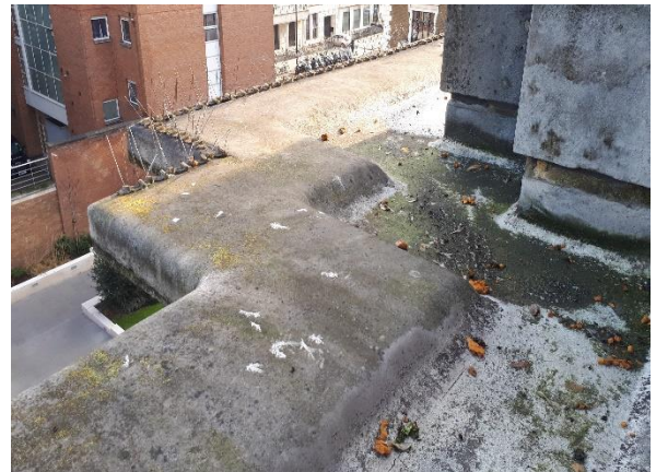
Existing asphalt finish on main cornice to external elevations showing gutter detail.
