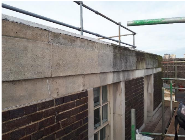
Cleaning to stonework at roof level. Photograph shows the difference between the soiled and clean stone.
