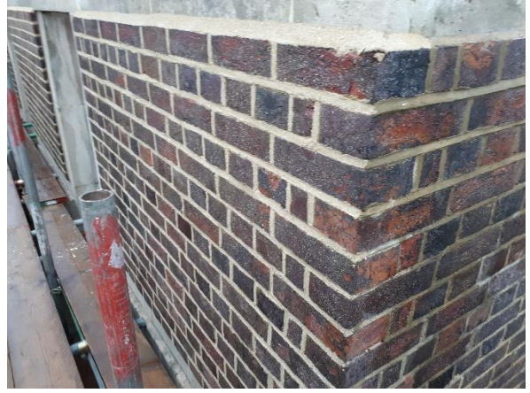
New pointing to external elevation.
