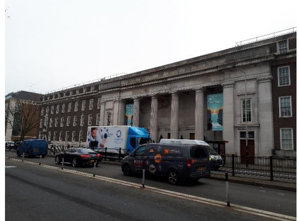
Euston Road elevation showing cornices at third floor level.
