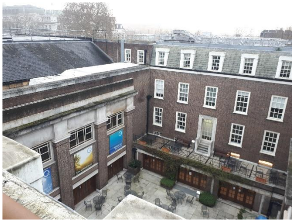
Existing asphalt finish to brick edge detail at third floor level to south-west elevation within the courtyard.
