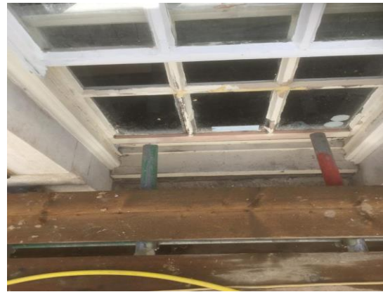
Example of putty repairs to sash windows.
