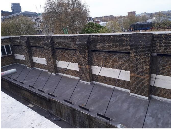
View of rendered panels to the brickwork wall within Roof 1.
