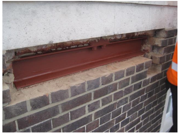
Treated steelwork behind brick panel.
