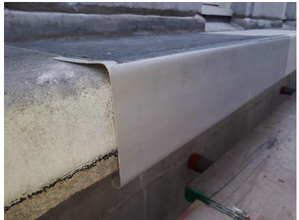
Photograph showing the profile of the proposed drip detail to the edge of the cornice.
