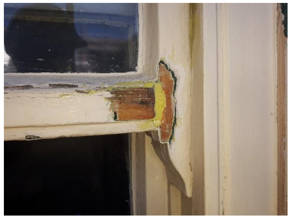
Epoxy resin repair to decayed conservation joint.
