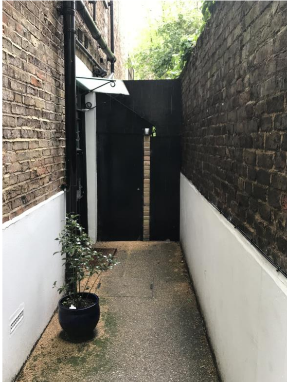
Fig 1 – Side passage way viewed from front of site
