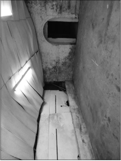
Internal Image of Unit 87
