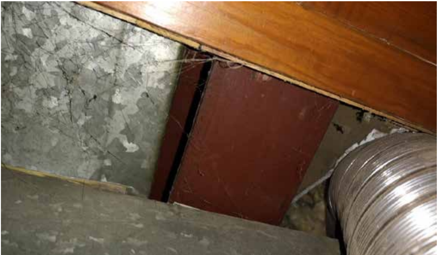
Figure 4: Existing metal beam in the basement
