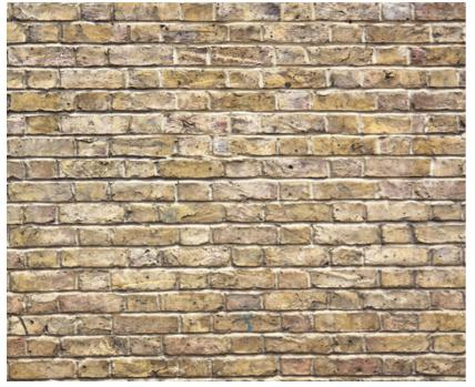
It is proposed that the extension be built from London Stock Brick to match the existing building. This is inline with the preapplication advice we received which advised that we should "consider a lightweight design or brick to match existing."
