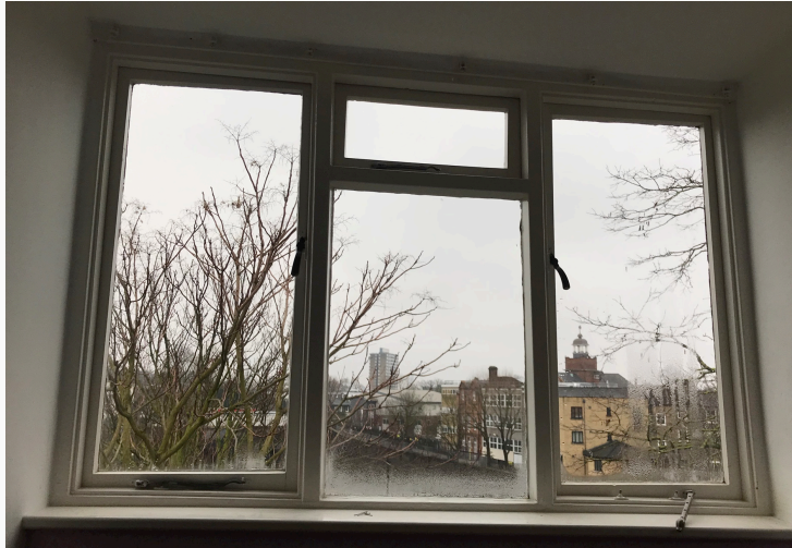
Existing single glazed window
