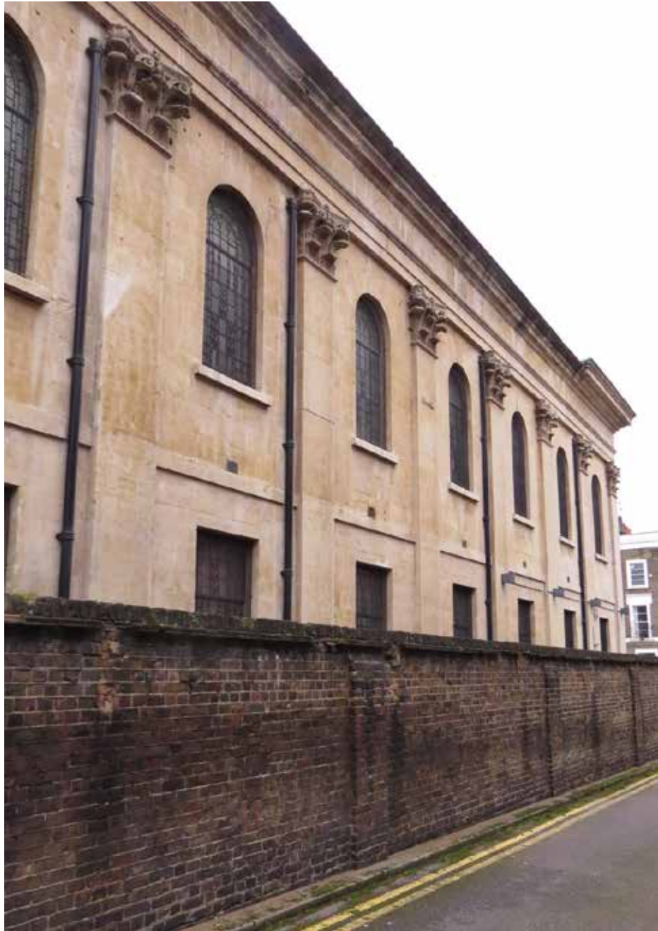
Figure 4.3 View of the west façade of the former Methodist Chapel
