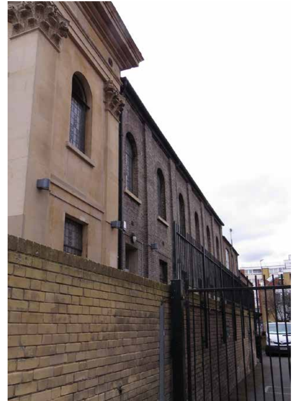
Figure 4.2 View of the east façade of the former Methodist Chapel
