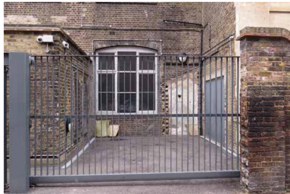
Figure 4.5 View of the rear access to the Building in the Middle Gallery
