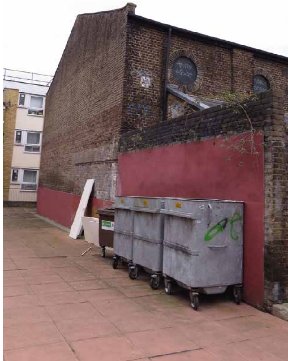
Figure 4.7 View of the rear façade
