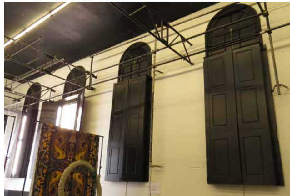
Figure 4.16 View of the rear gallery space
