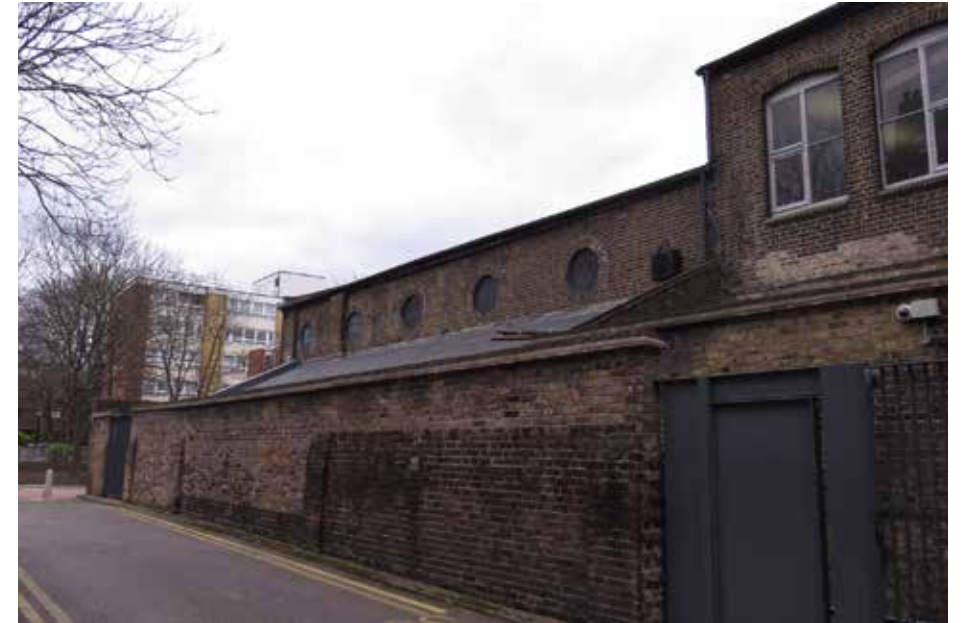
Figure 4.6 View of the west return of the former Methodist Chapel, the rear and middle gallery
