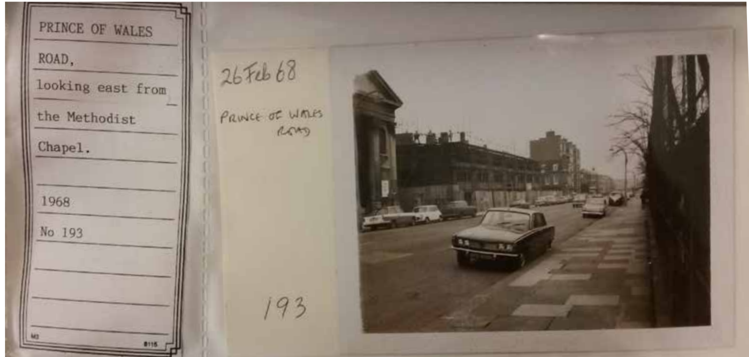
Figure 3.8 View of the former chapel in 1968, with the neighbouring building during construction
