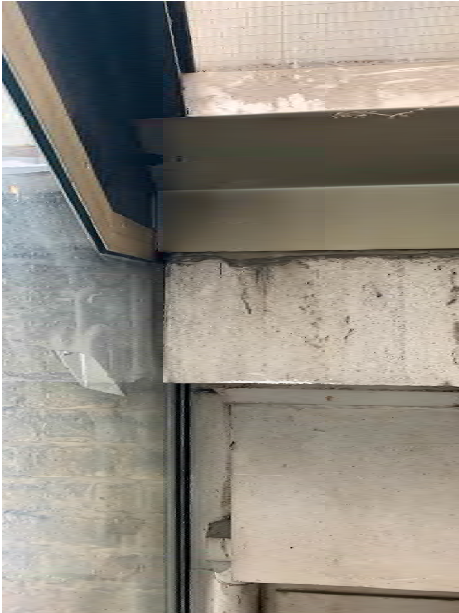
Figure 2: Detail of aluminium structure and glazed walls connected to Lethaby Building
