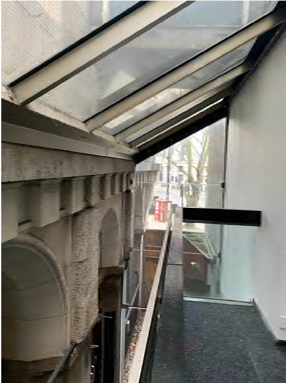
Figure 3: Showing roof connection of glazed link to historic fabric of Lethaby Building
