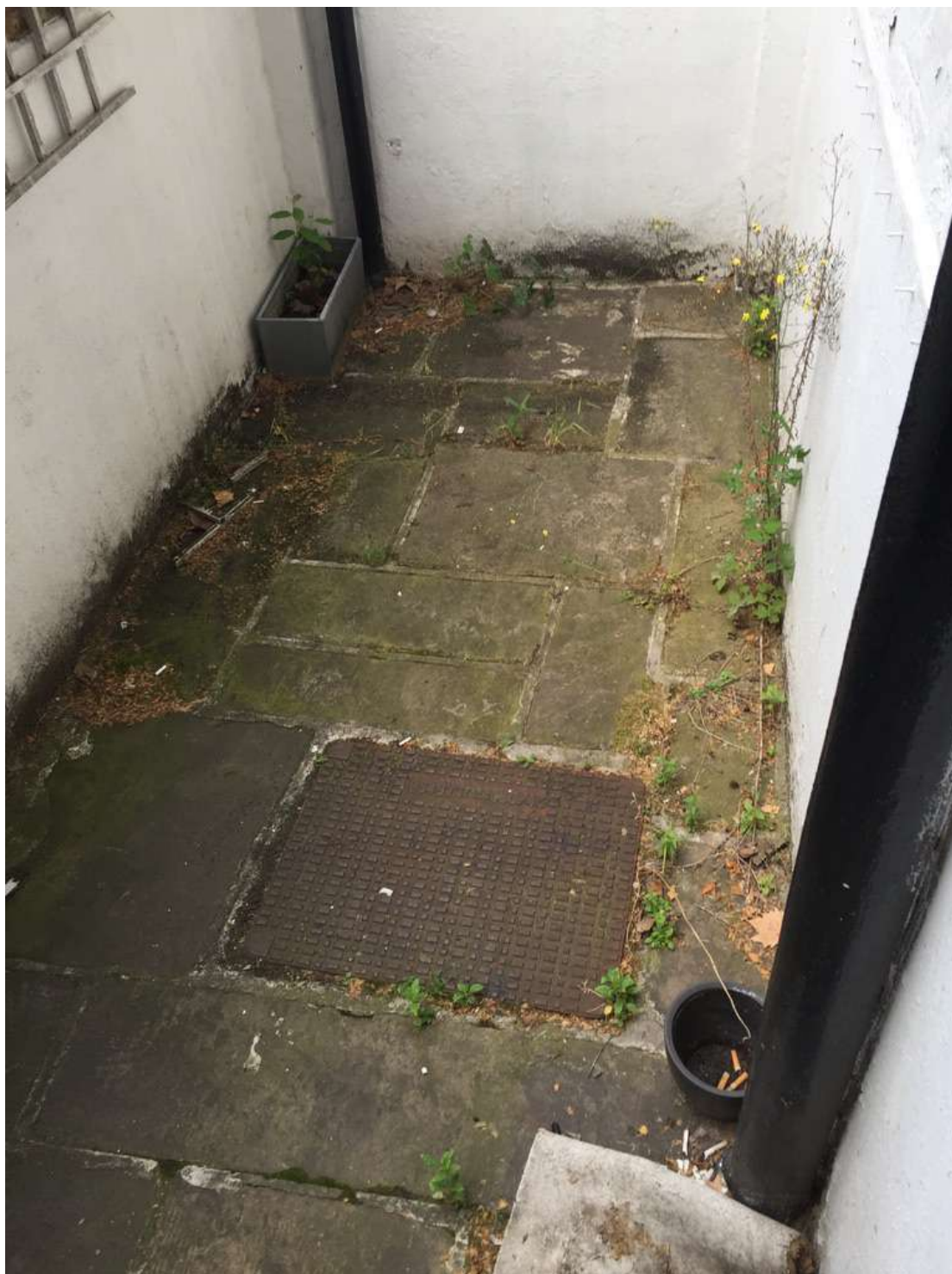
Stone flag floor to the rear yard has been laid around the modern drain cover.
