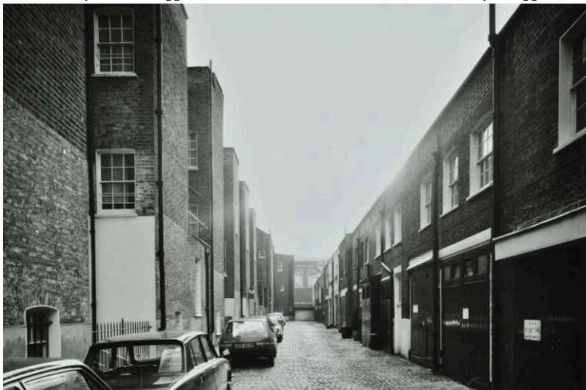
Gloucester Gate Mews in 1981 looking north and south. Note (above) the truncated outrigger at No 205 only survives to first floor half landing level. The single storey extension is also in place and has a traditional rainwater hopper. Looking south (below) shows the rhythm of outriggers with sashes in the flank of the more northerly outriggers.
