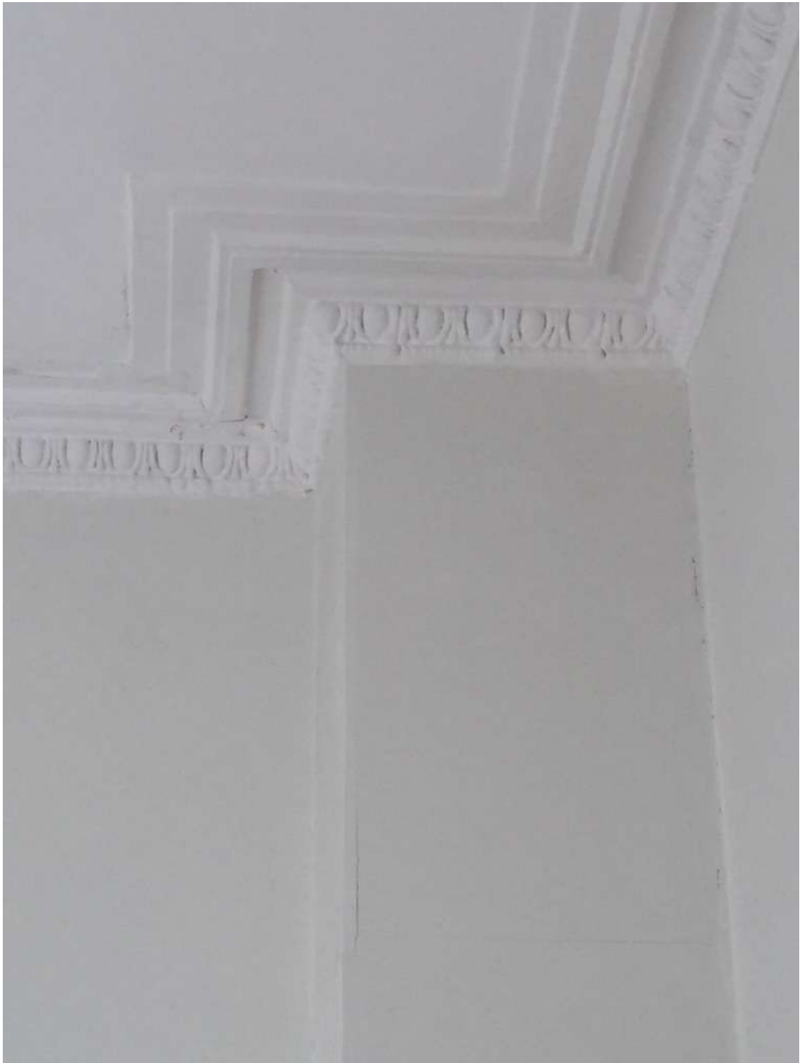
Ovolo cornice run around boxed in pipework in small first floor front room.
