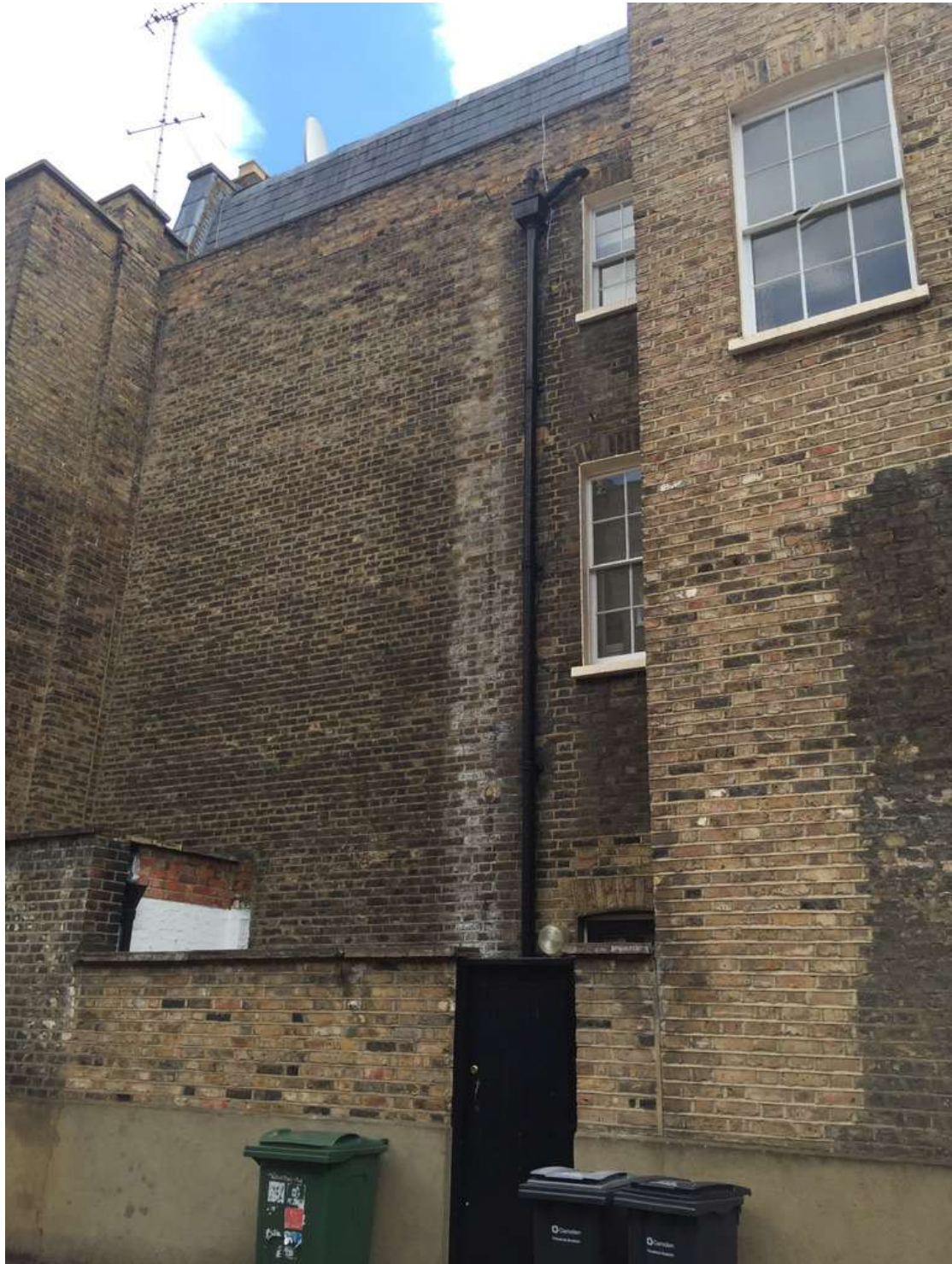
Rear of 205 with extensively reconstructed outrigger with modern sash and yard wall. The parapet below the mansard also appears to have been rebuilt. The yard wall is also modern (possible since the 1987 permission). The single storey extension is a patchwork of yellow stock brick, red brick and painted brick.
