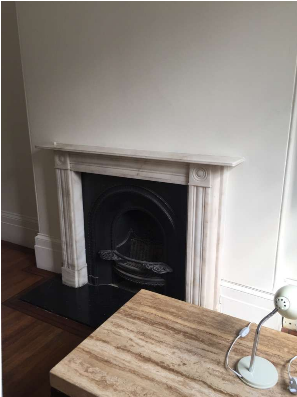
Marble mantle in the main room at ground floor. Much of the flat plaster appears to be modern.
