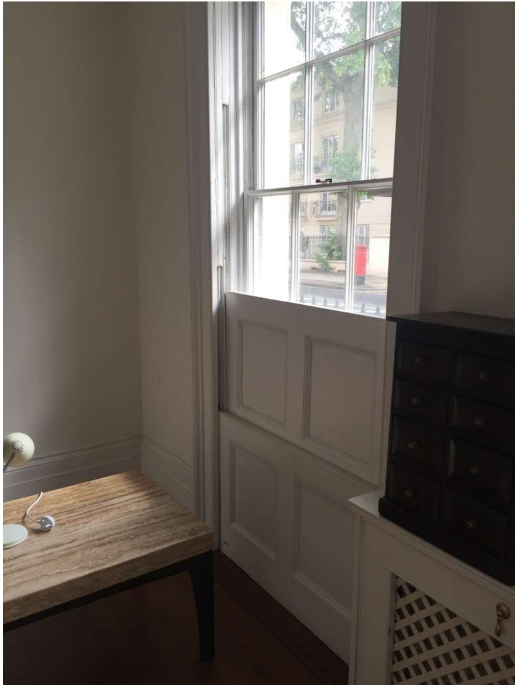
Detail of the main room at ground level: the shutters and window architrave appear original. The sashes are more recent and possibly the skirting.
