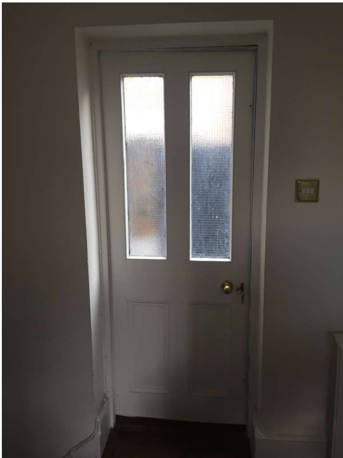
Back door to the rear yard. It is possible that this has been relocated from the outrigger flank (an arrangement on neighbouring properties) but the skirting arrangement appears original.
