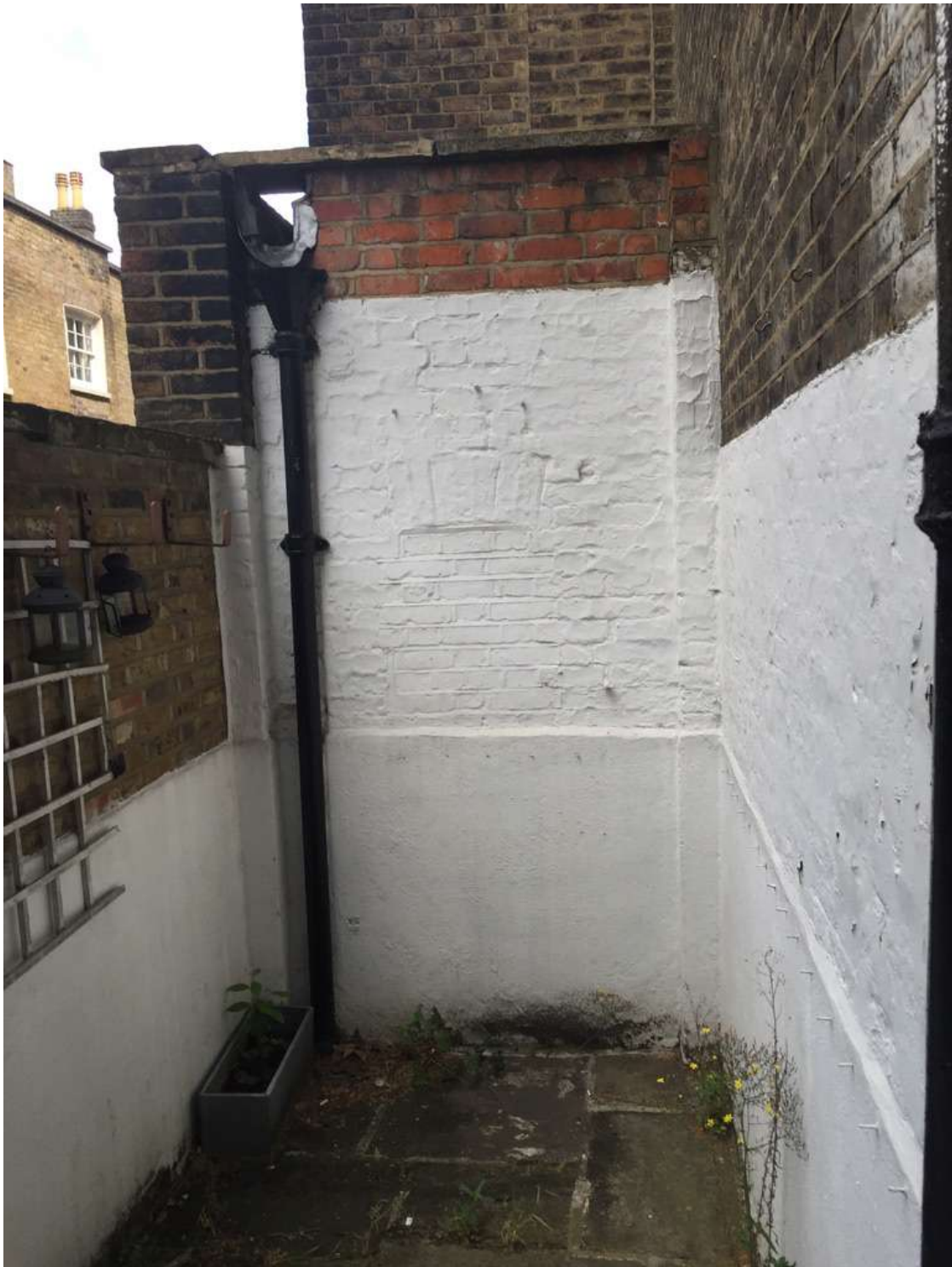
Rear yard looking to single-storey extension with modern boundary wall. It once contained a window between a brick arch and may once have contained a privy. The red brick upper part is 20 th century work.
