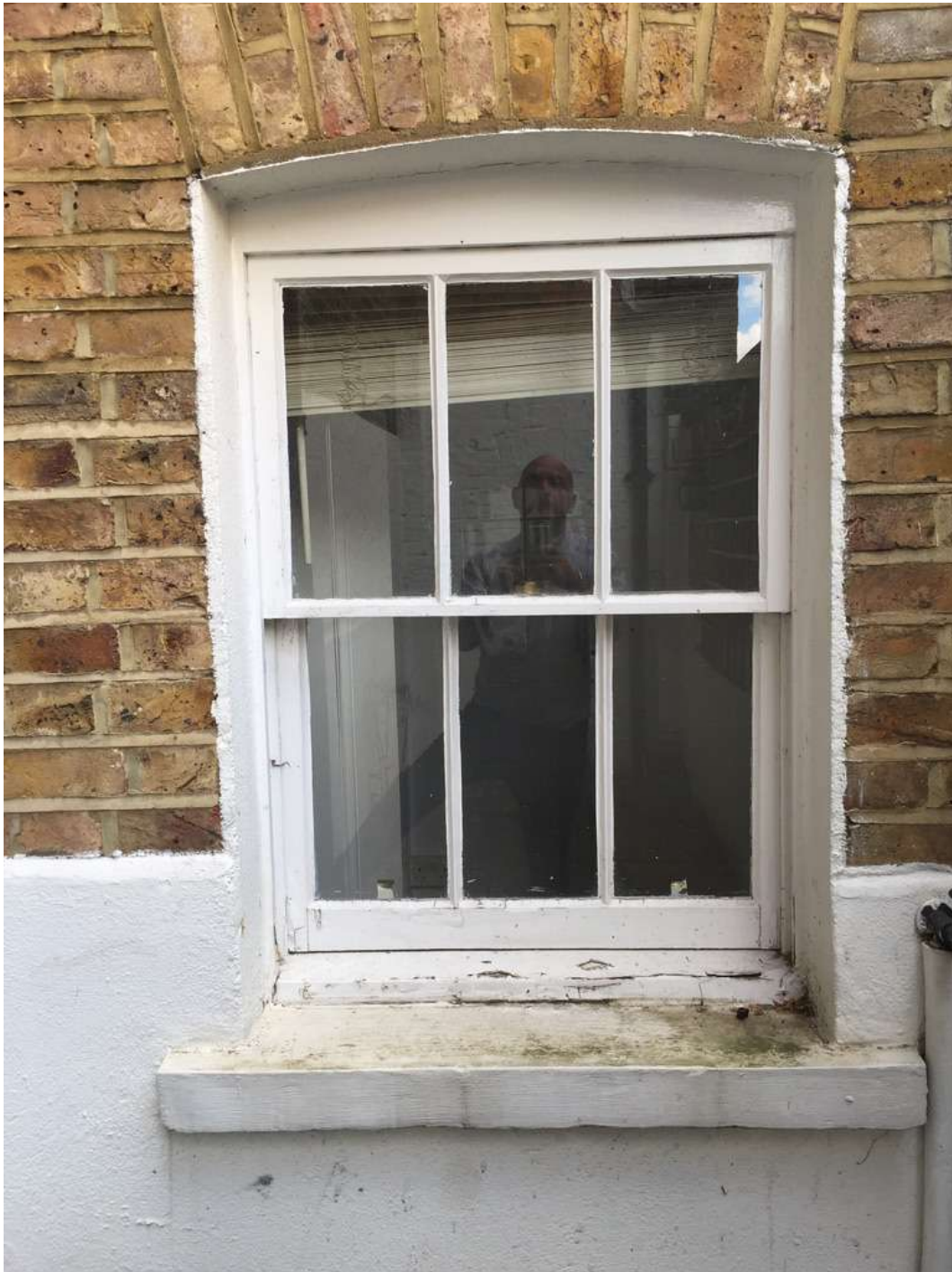
Modern sash window on the flank of the reconstructed outrigger.
