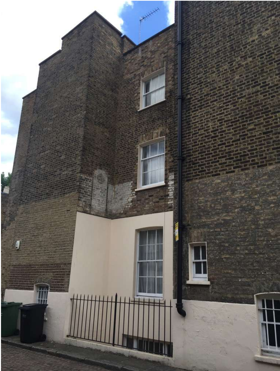
The rear of 217 with a different yard arrangement again – perhaps the original arrangement – but with sash windows at upper level as well as ground.
