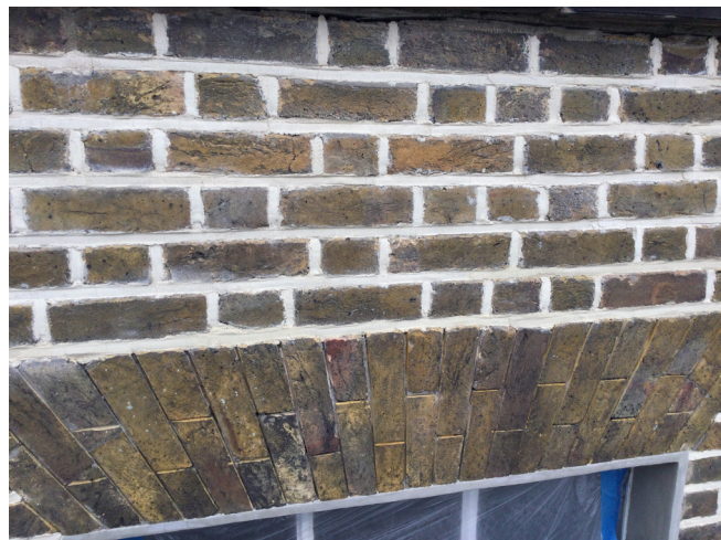
Figure 4: Repointing to upper lift
