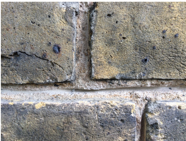
Figure 3: Typical detail of mortar removal
