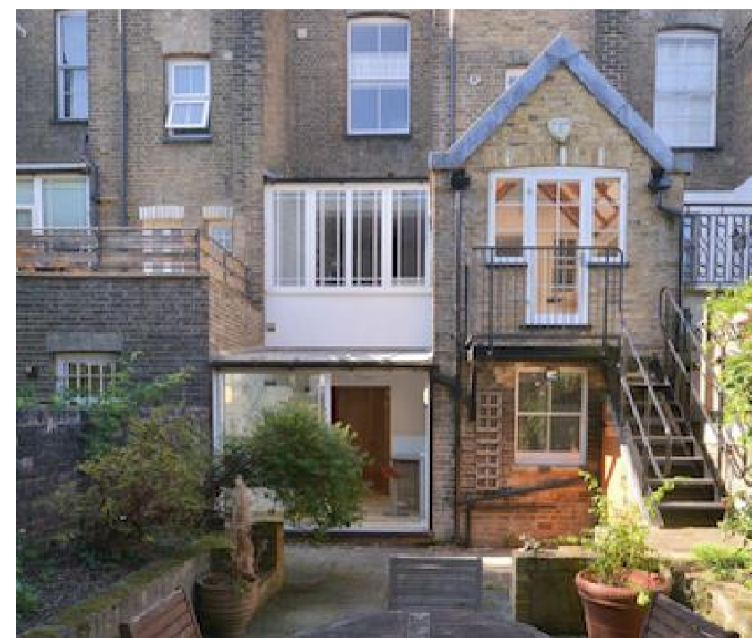
SITE PHOTOGRAPH REAR ELEVATION (LOWER FLOORS)
