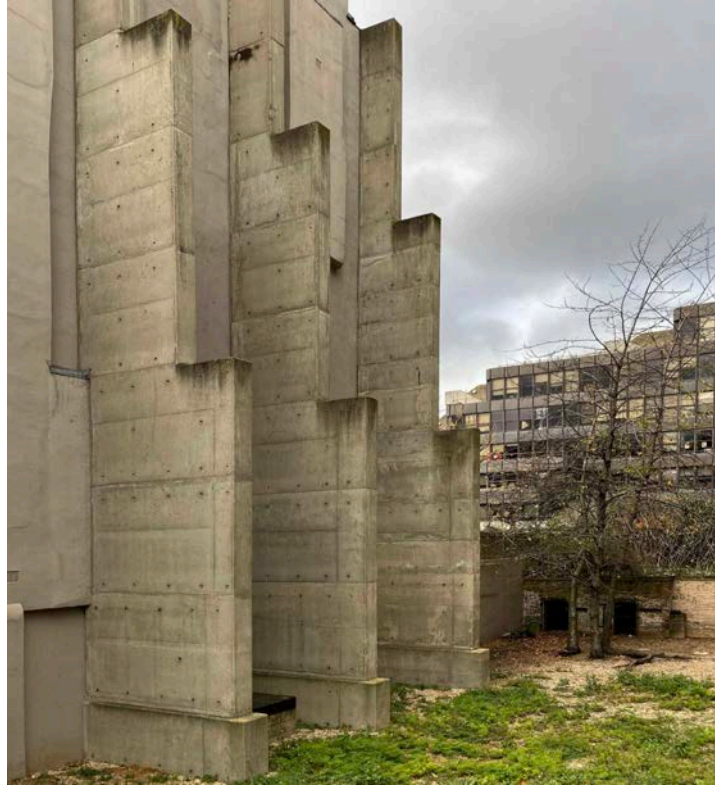
Figure 20 Reinforced concrete buttresses propping the party wall of No. 21 Russell Square. (Nick Collins).
