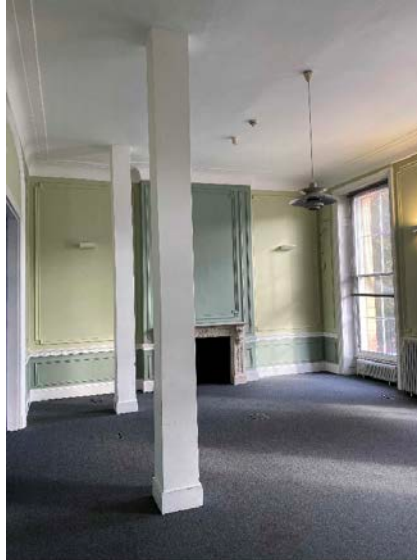
Figures 25 & 26 An office in No. 24 as restored and altered in the late 1990s, and in 2020. The slender square-section columns were probably introduced in the 1990s, although conceivably they date from c1935, when Lander, Bedells and Crompton made alterations to the building. ( www.circmanagement.com/Nick Collins ).
