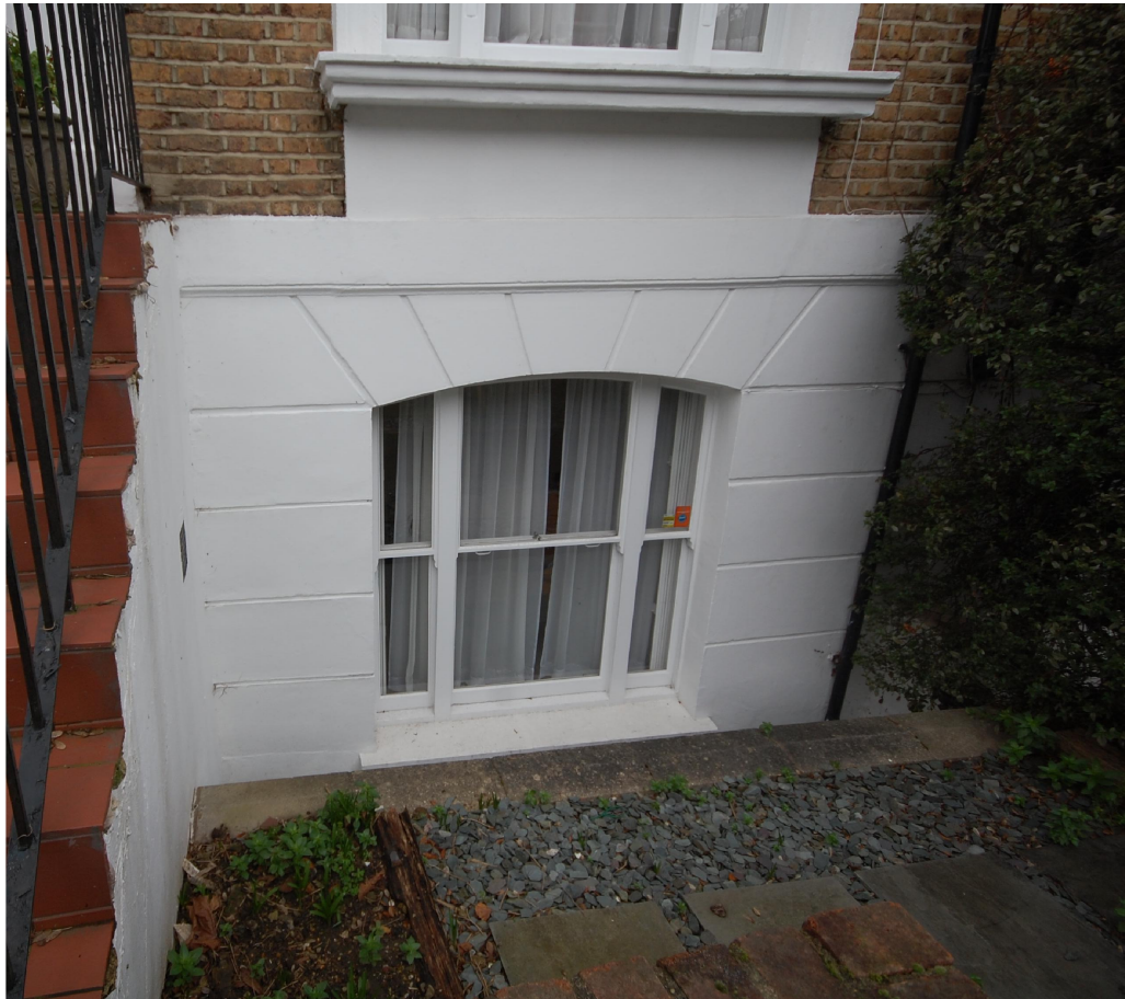
FRONT ELEVATION - EXISTING LIGHT-WELL TO BE DEEPEMED
