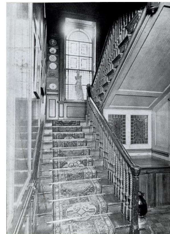
Detail of the early 18 th century staircase: panelling, handrail and balustrading
