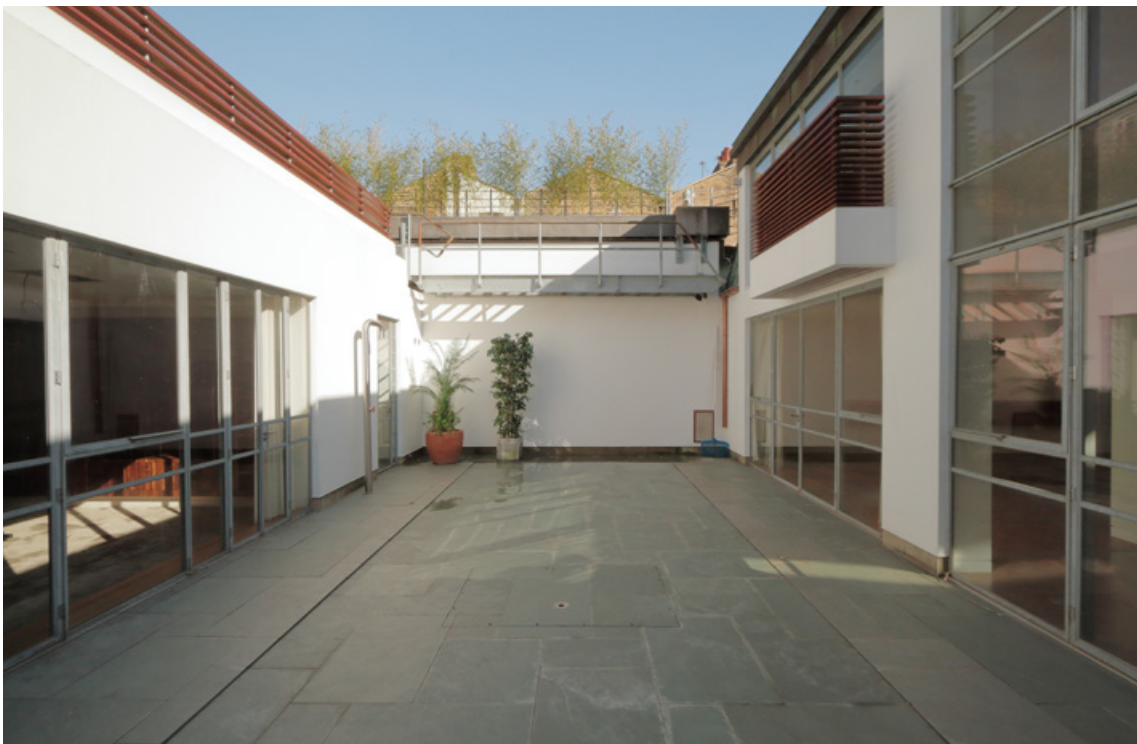
[B] View of existing pool courtyard, due south-east [image source: Author]
