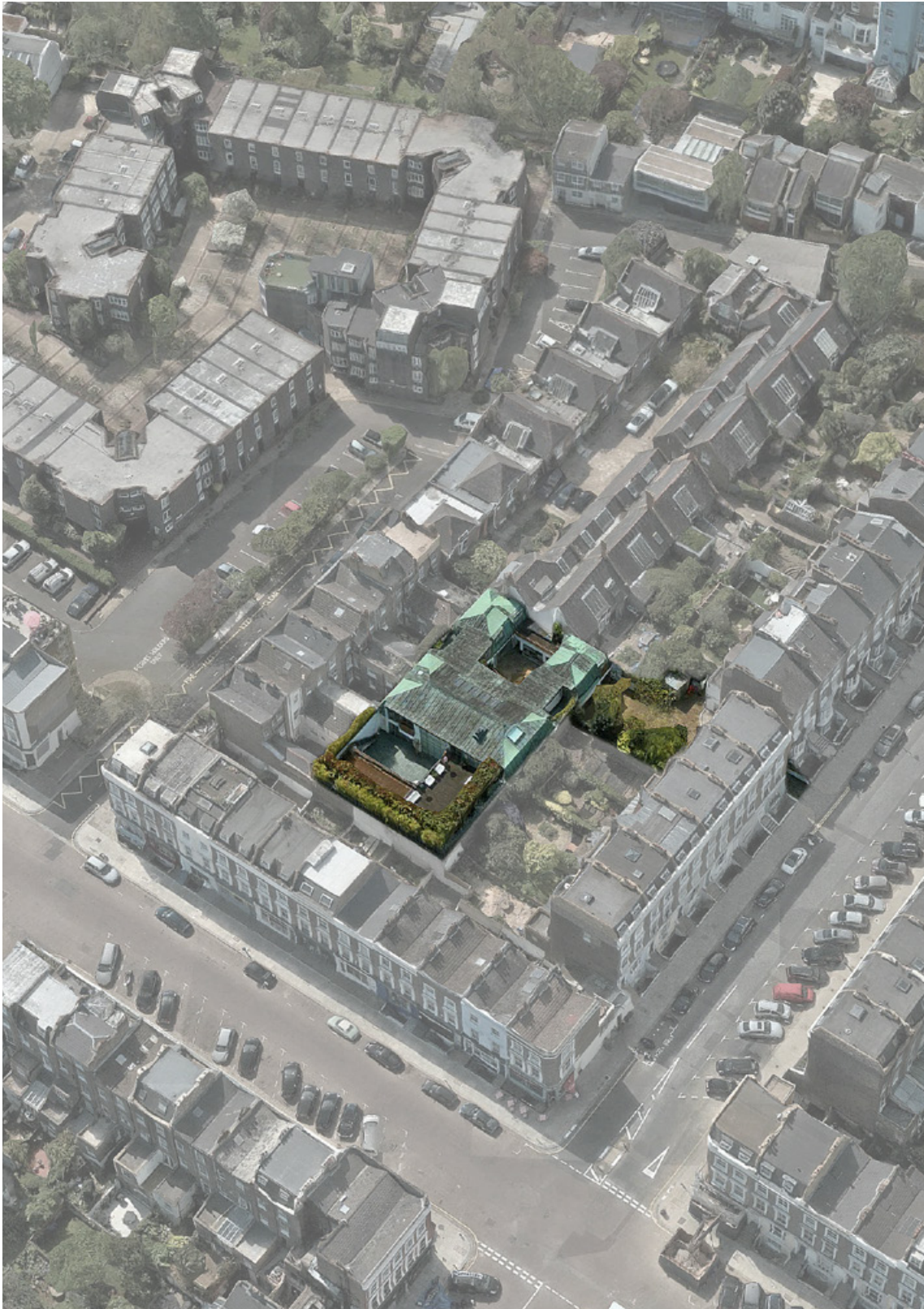
Aerial photo showing site and context looking due south [image source: Apple Maps]
