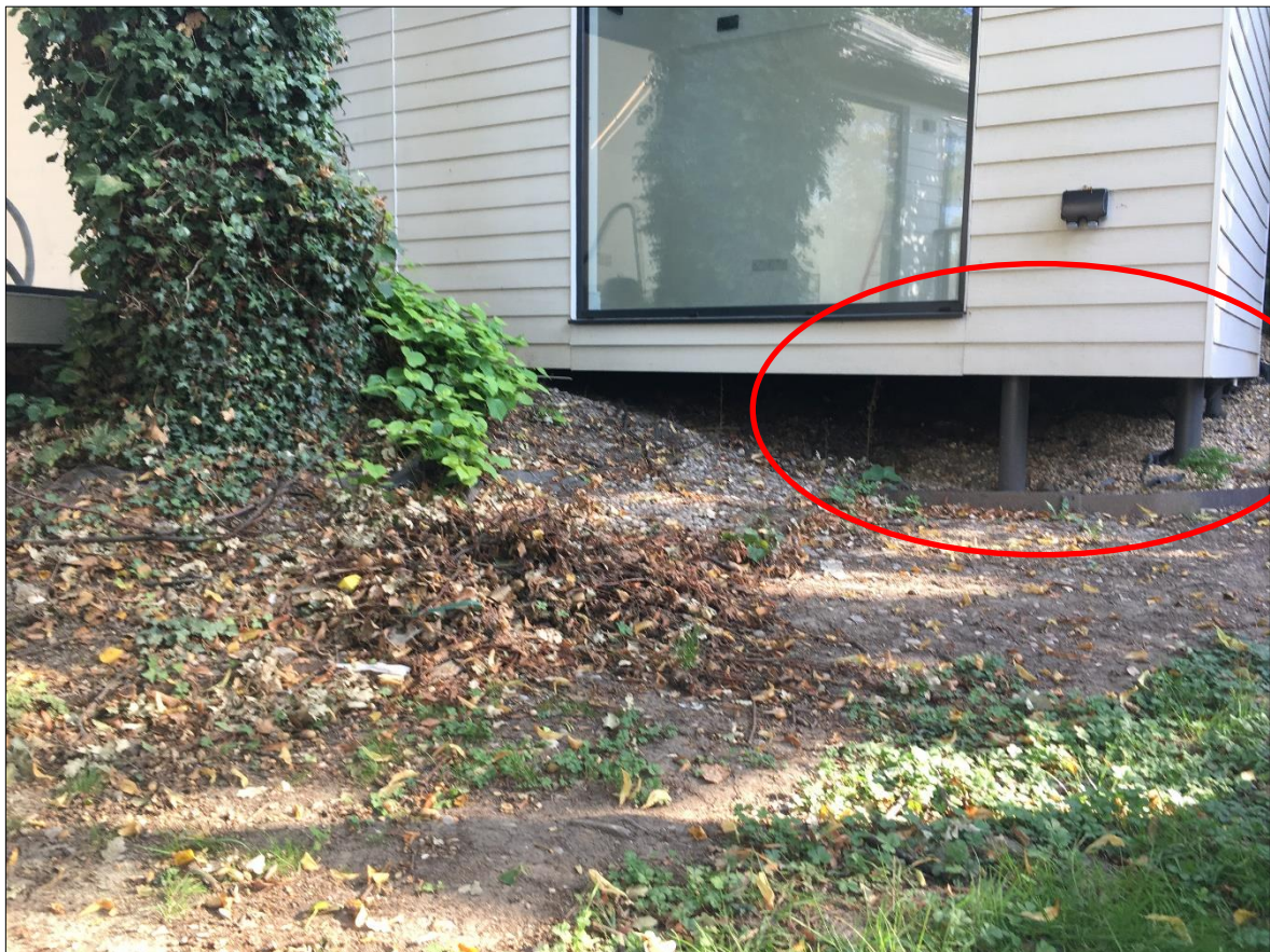
Fig. 2 Example of micro piles in use for an out building (Hampstead 2018)
