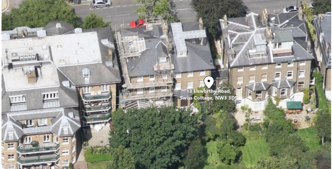
Figure 2: The roofscape context of the Site (Bing Maps)
