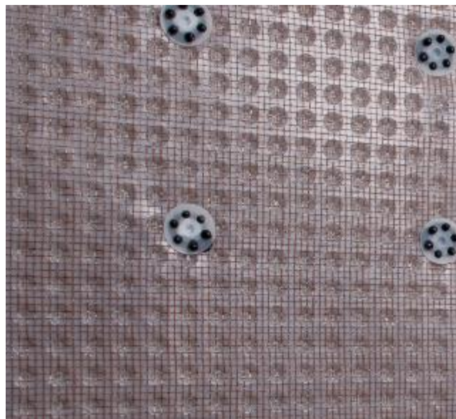
Figure 3: Example of dimpled membrane used for waterproofing basements
