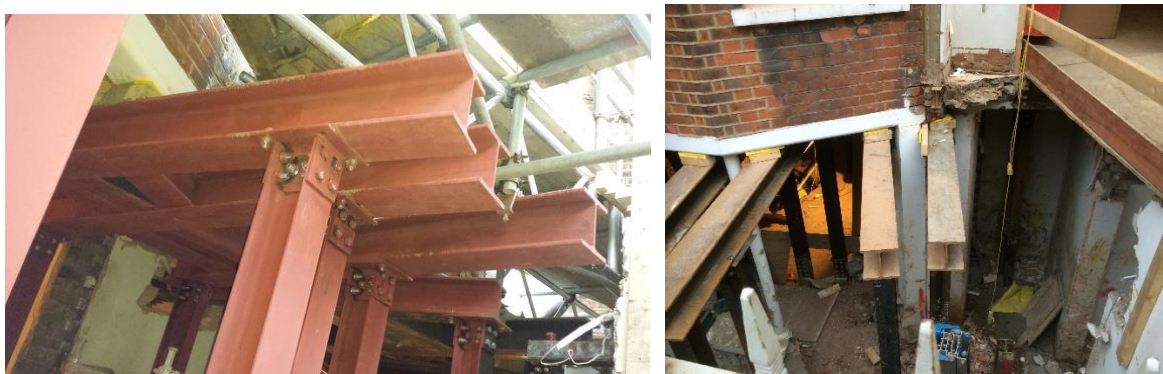
Figure 1 Example of needling to existing wall
