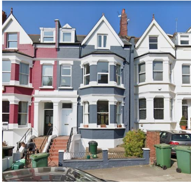
Figure 3 - view on front elevation, 15 Lyncroft Gardens
