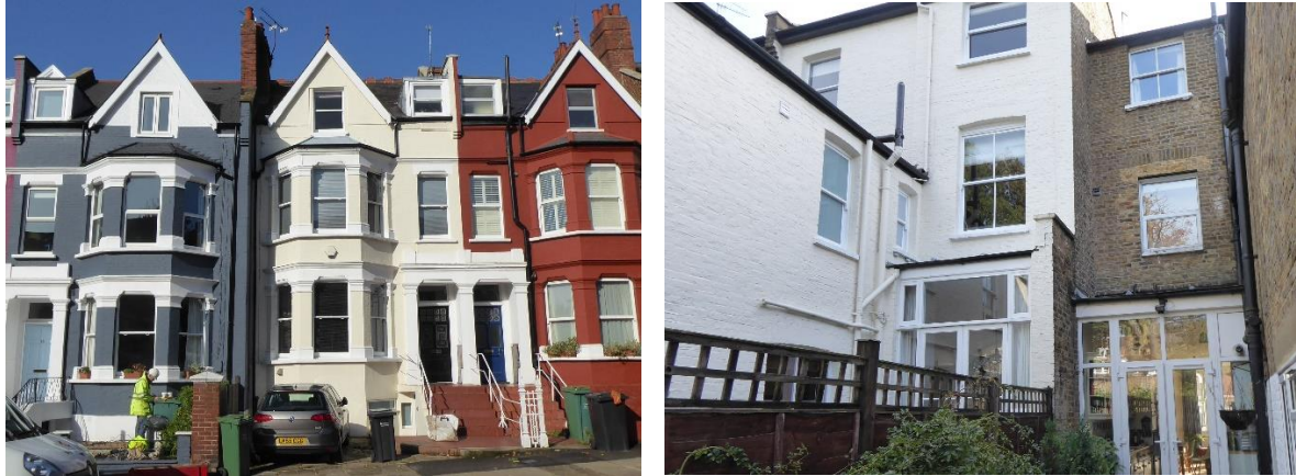
Figure 5 View on front and rear elevations, 17 Lyncroft Gardens
