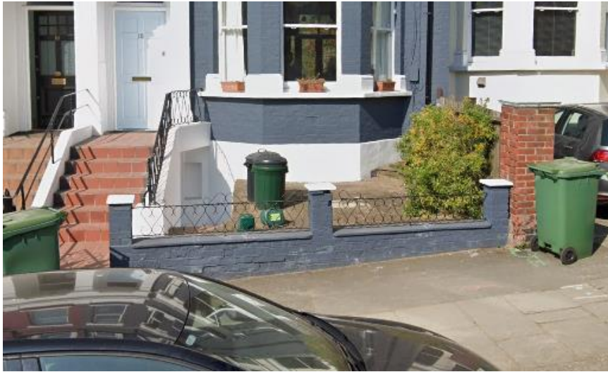
Figure 2: Passive Defences at 15 Lyncroft Gardens
