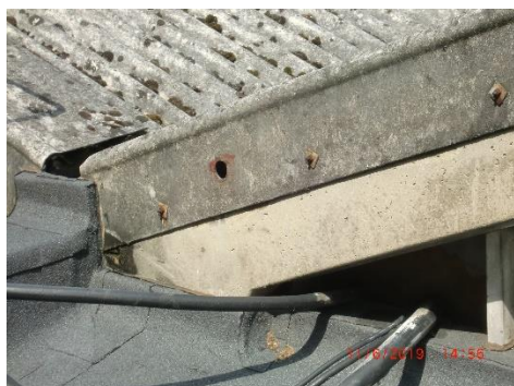
Photo 7: Small hole in edge of roof of B4.
