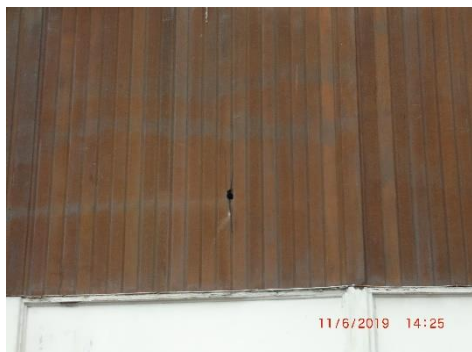
Photo 5: Small hole in northern elevation of B2
