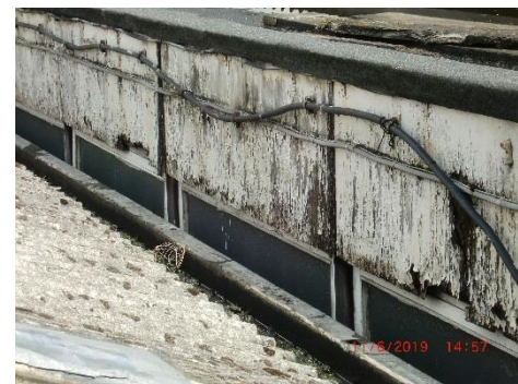
Photo 6: Cracks in wall of B2 (west facing)
