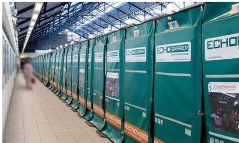
Figure 5: Lightweight barrier with sound panels
