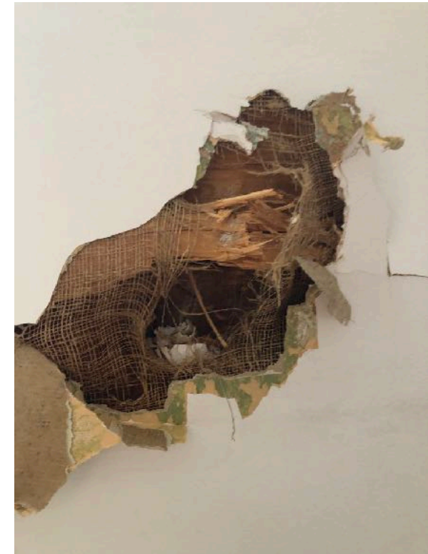
An investigation hole undertaken to the wall showing a void between wall line and brickwork
