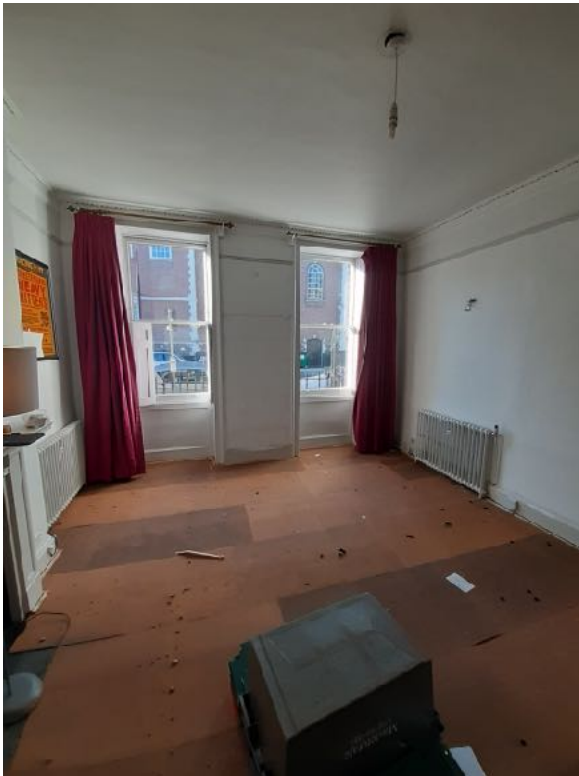
Upper Ground Floor front room showing evidence of damp between windows
