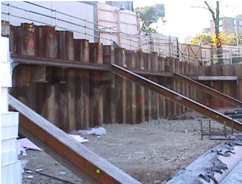
Figure 6-2 Propped sheet piled wall
