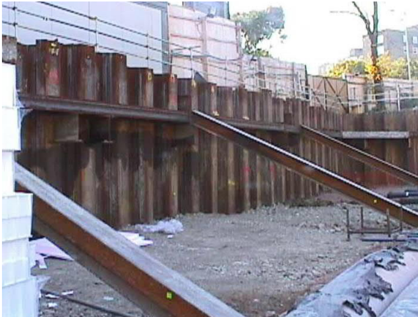
Figure 6-2 Propped sheet piled wall
