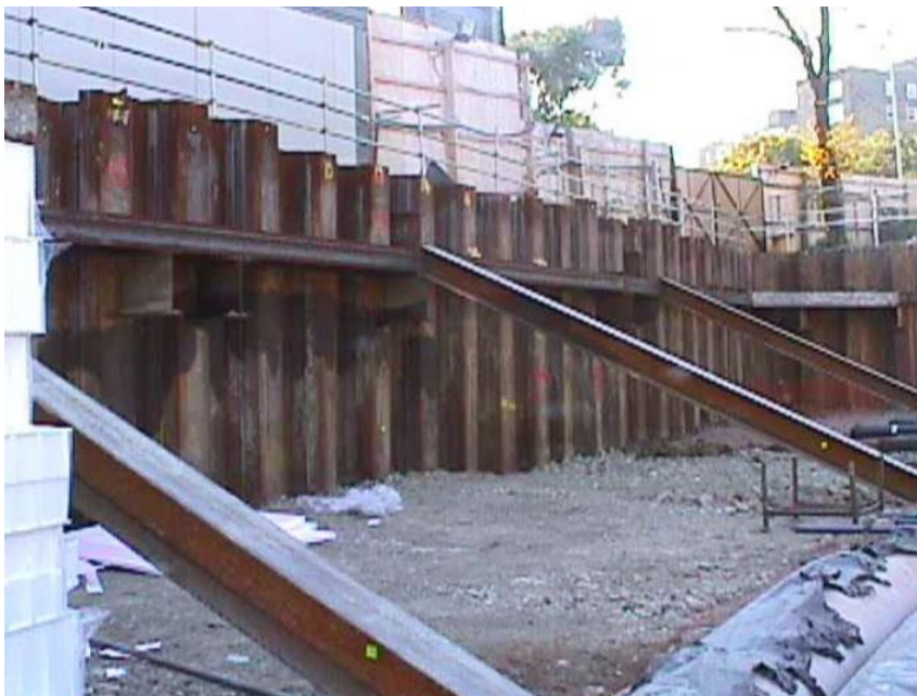
Figure 6-2 Propped sheet piled wall
